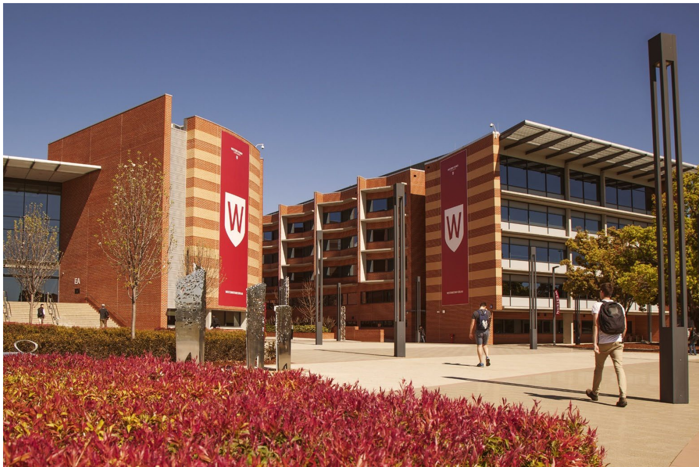
Figure 12 EA and EB buildings
