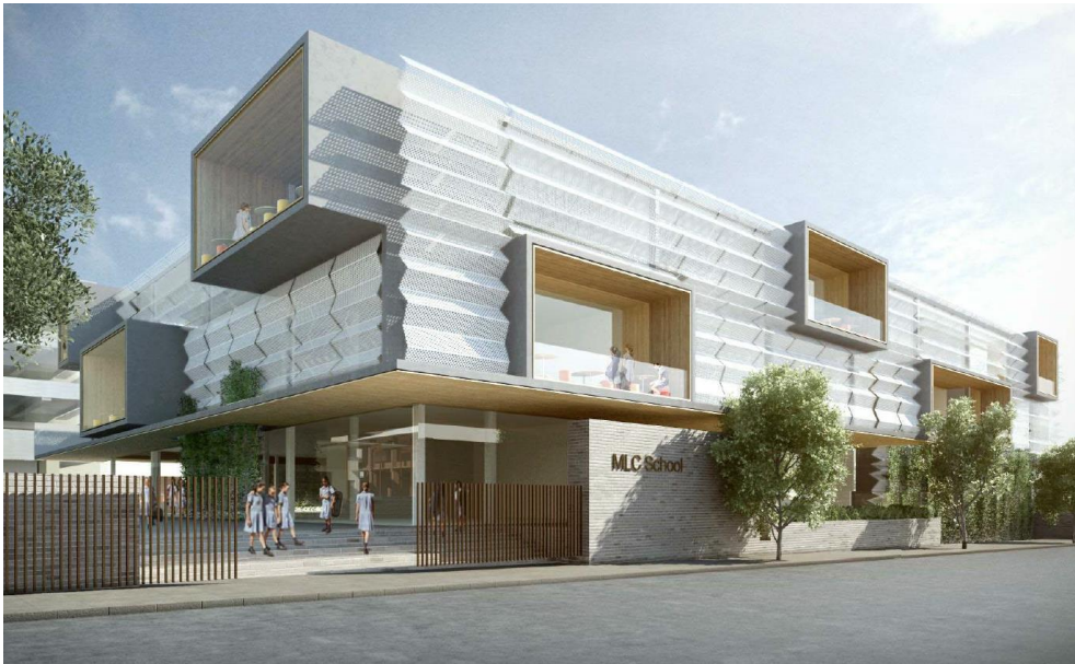
Figure 3 – Approved Teaching and Learning Building (Main Building) viewed from Park Road
