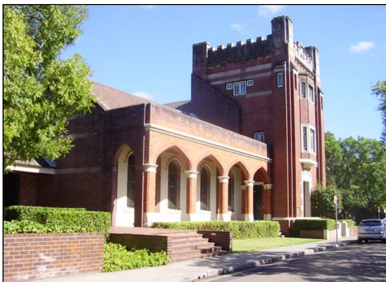
Figure 3.33 The most significant features of the site are located in the southern section near the Rowley Street frontage. The Schofield Tower and Chapel are the oldest buildings on the site and survived the 1977 fire. The single storey Chapel was constructed in 1891-92. The Tower and associated wing were constructed in 1919.
