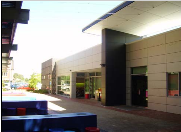
Figure 3.58 The Middle School was constructed in 2010.
