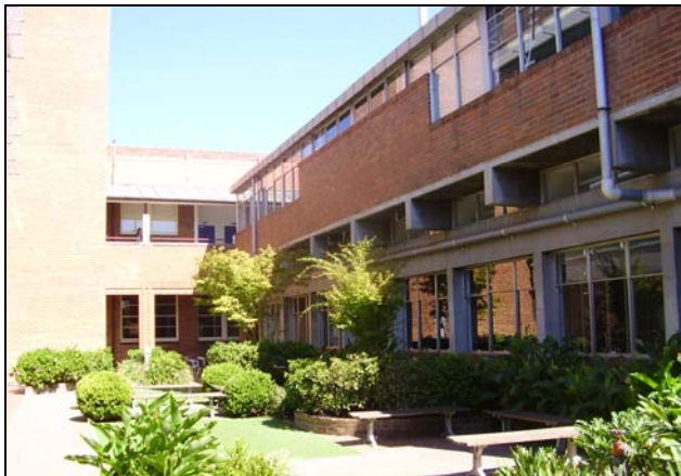
Figure 3.45 The southern facade of Building 10 which was constructed in 1960. It is a simple utilitarian building constructed in concrete and brick with parapeted flat roof and aluminium framed windows.
