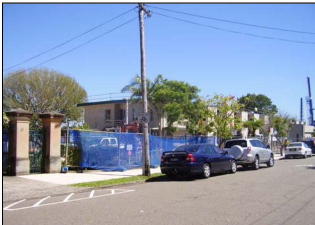
Figure 3.24 The St John of God Hospital. Construction works, alterations and additions to the building are currently in progress.
