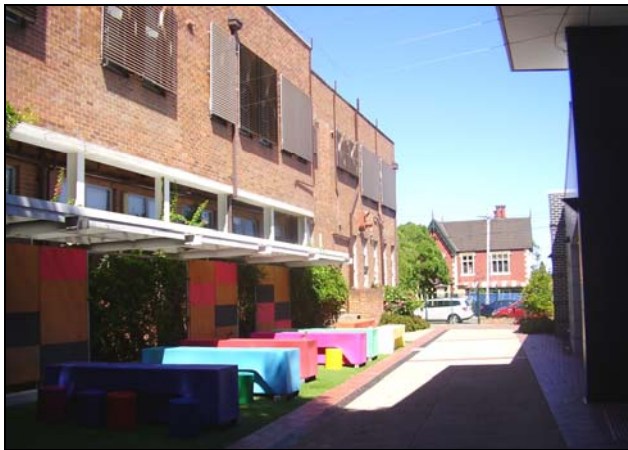
Figure 3.63 The open space between the Middle School and Buildings 10 and 11.
