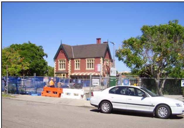
Figure 3.23 Grantham , (No. 21 Grantham Street) is a large two storey Victorian Gothic style former dwelling. The building has been listed as an item and is also part of the St John of God complex. The building is set well back from the street frontage with garden and driveway located between.
