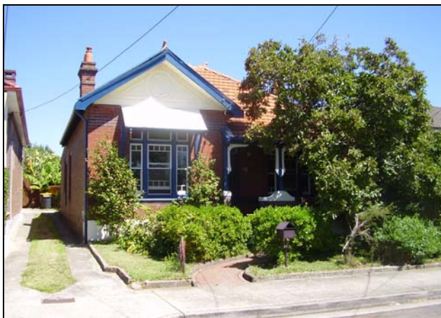
Figure 3.11 No. 31 Park Road is a single storey face brick with rendered base Federation period cottage with gabled and hipped main roof clad in terracotta tiles. The building is setback from the street frontage with small planted garden between. An open driveway extends along the southern side boundary to a detached garage located the rear of the house.
