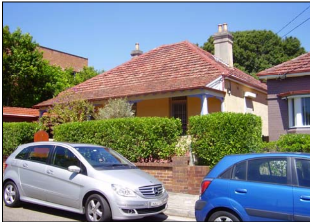
Figure 3.52 Two residential properties and cottages to the north of the School site have been added to the School site. No. 33 Park Road is a single storey painted brick modified cottage with hipped tiled roof and open front verandah. A small carport has been added to the site (just visible at left)
