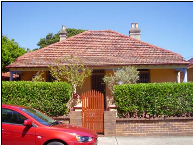
Figure 3.53 No. 33 Park Road.
