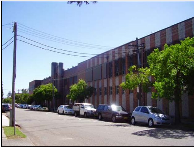
Figure 3.68 The buildings along Grantham Street. Building 7, with distinctive striped façade (mid hot) was constructed in the early 1960s.
