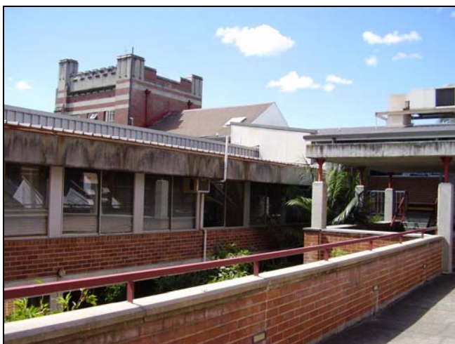
Figure 3.43 Part of Building 17 (at left) from the elevated walkway (15 on site map).
