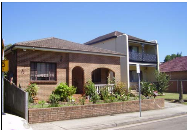
Figure 3.12 No. 29 Park Road is a modified face brick single storey dwelling with hipped roof clad in tiles. The building is also setback from the street frontage with small front garden and open driveway extending along the northern site boundary.
