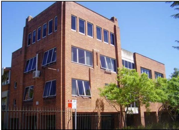
Figure 3.49 The New Tower and Building 12 which was constructed in the 1990s.
