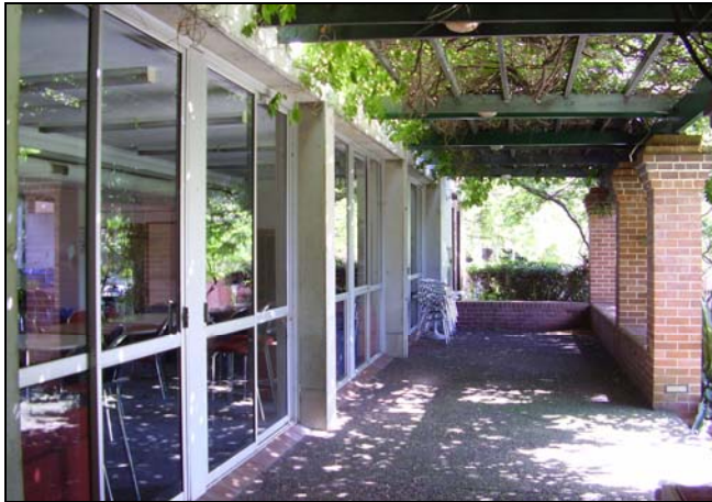
Figure 3.41 The building extends in a north-south orientation from the junction of the Schofield Tower and Building 4. The eastern façade, which faces the Principal's Lawn and Park Road frontage features an open verandah with pergola supported on heavy brick piers.
