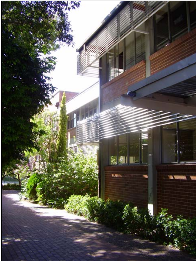
Figure 3.51 The northern facade of Buildings 11 and 12.
