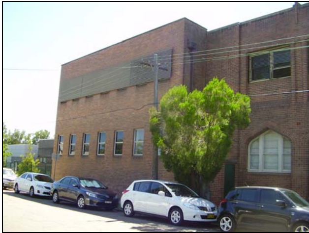
Figure 3.65 The Grantham Street façade of Building 10. The face brick façade is simple and utilitarian and is constructed to the 1940s Sutton Wing.
