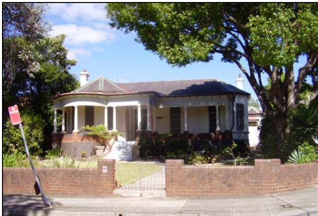
Figure 3.3 The building, No. 47 Park Road has been listed as an item and has mature trees and plantings along Rowley Street frontage.
