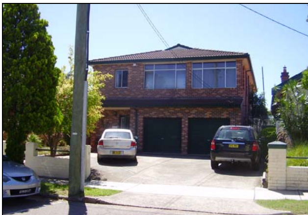
Figure 3.28 The buildings along this section of Grantham Street generally date from the 20 th century and include some modern two and three storey infill development.
