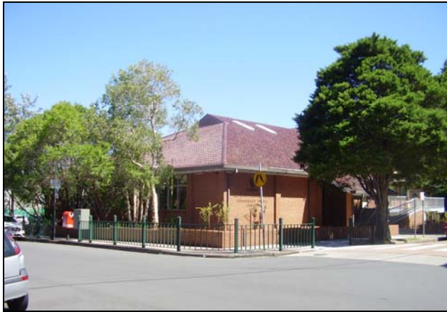
Figure 3.18 The School buildings including the 1980s Centenary Music Centre occupy the southern part of the street.
