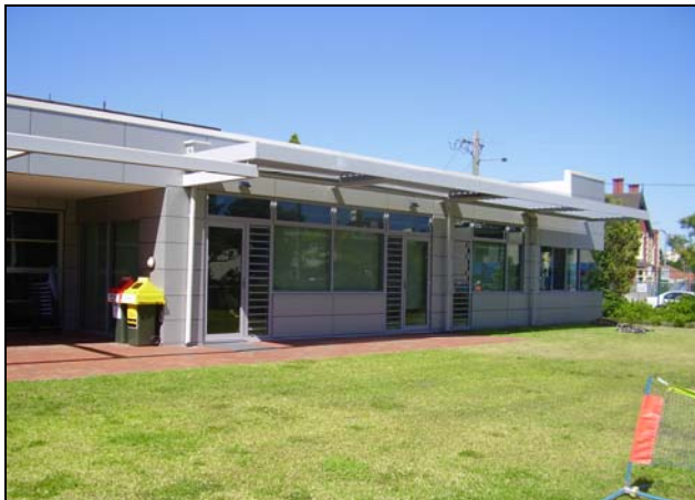
Figure 3.60 The northern façade of the building faces and open lawn.
