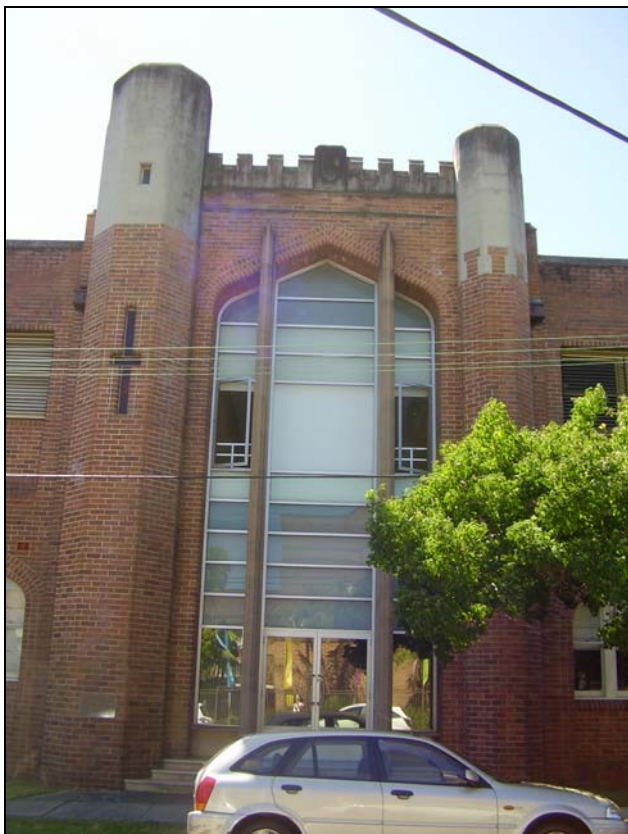
Figure 3.67 A notable feature of the Grantham Street frontage is the former entry to Building 9, the Sutton Wing, which was constructed in the late 1940s.
