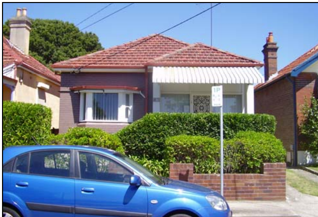
Figure 3.55 No. 31A Park Road (Building 14 Site Map) is also a modified painted brick cottage with hipped roof clad in terracotta tiles.
