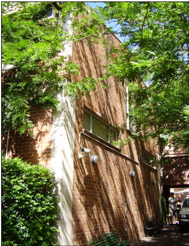
Figure 3.42 The building is also a simple building with expressed concrete framing, low pitched gabled roof and aluminium framed windows.
