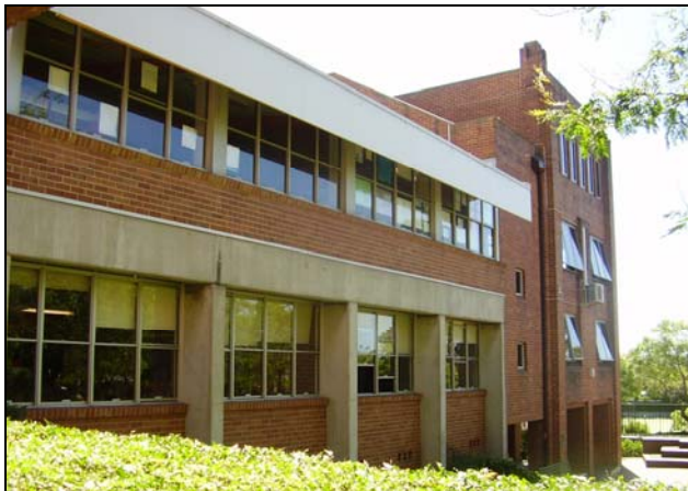
Figure 3.46 Building 11 is a two storey brick and concrete building constructed in the 1980s. The building was constructed to Building 10 and was also extended in the 1990s when the new Tower classrooms and Tuckshop (Building 12) was constructed at its eastern end.
