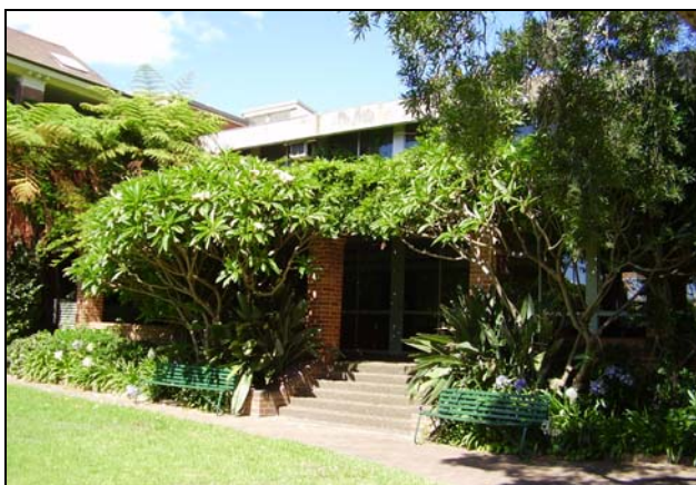
Figure 3.40 Building 17 is a two storey face brick, concrete and glass building.
