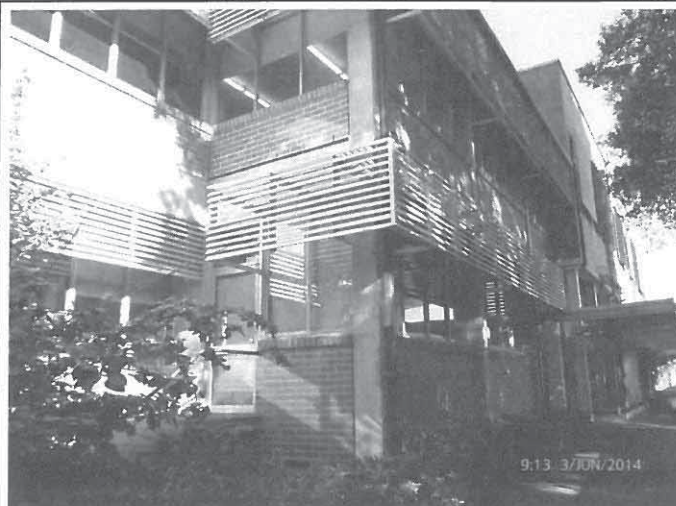
Photograph 2 – Looking south west at building on southern portion of the site.
