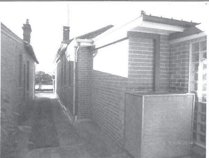
Photograph 6 – Looking east down the driveway located on the northern side of site
