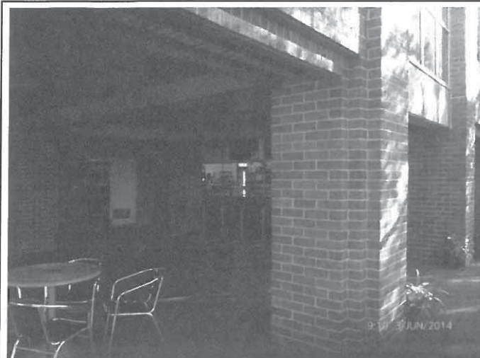
Photograph 1 – Looking south west at the school canteen underneath the building on the southern portion of the site.
