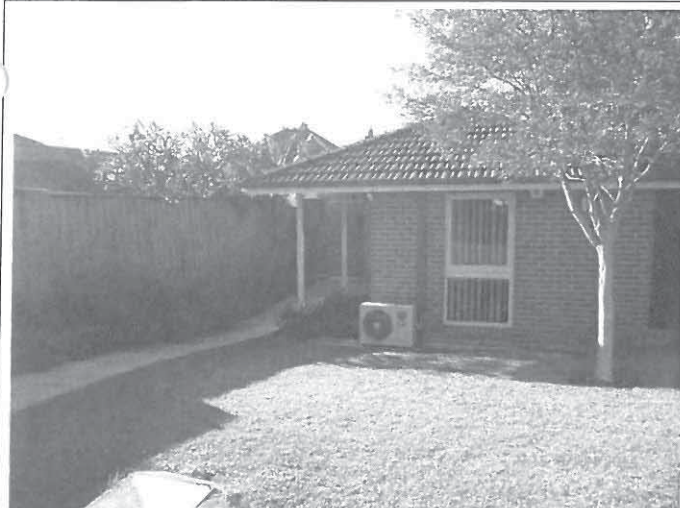
Photograph 7 – Looking north east at the backyard of the house located at 31A Park Road
