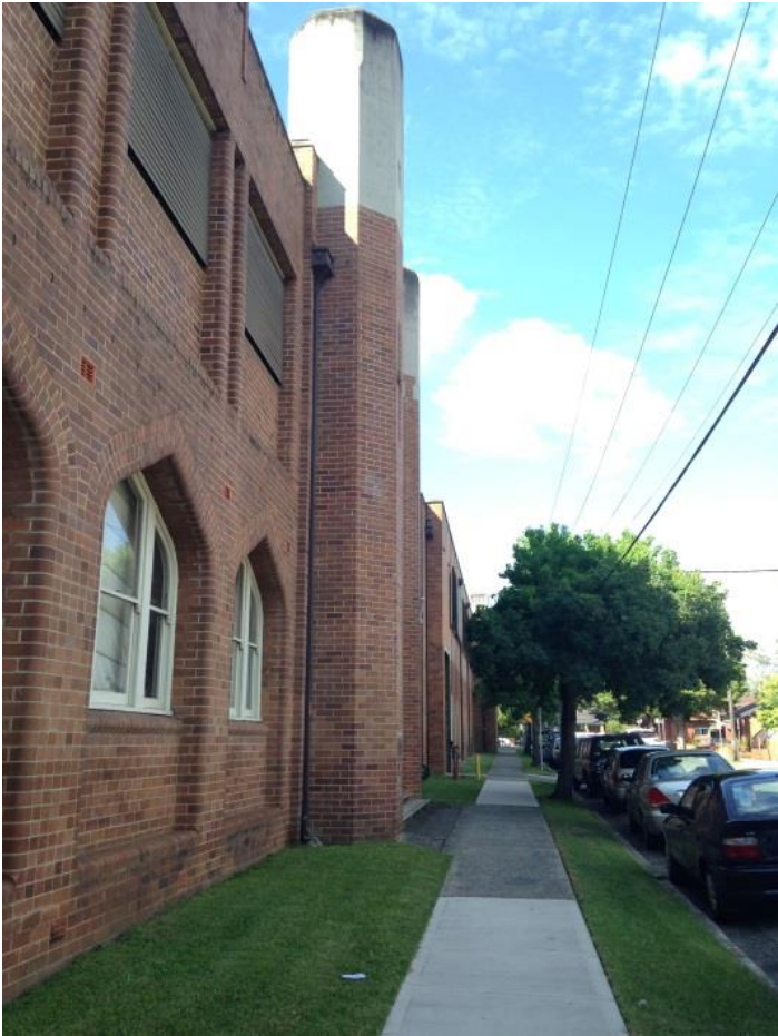
Figure 9 – Sutton Wing and Wade House along Grantham Street Source: JBA
