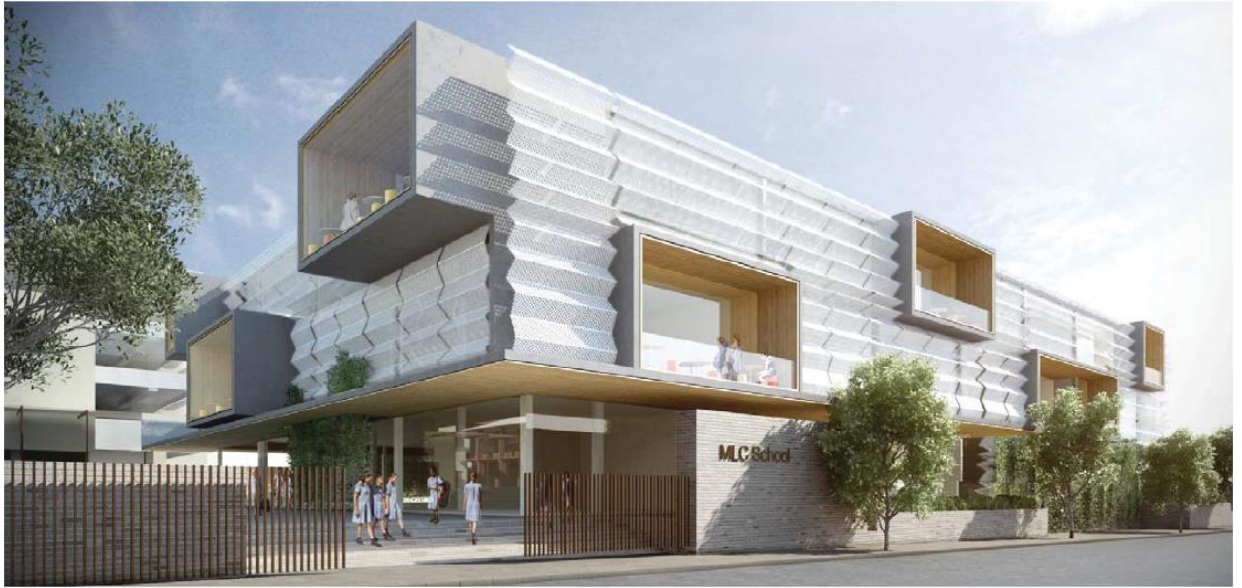
Figure 20 – View of the main building from Park Road Source: BVN Donovan Hill
