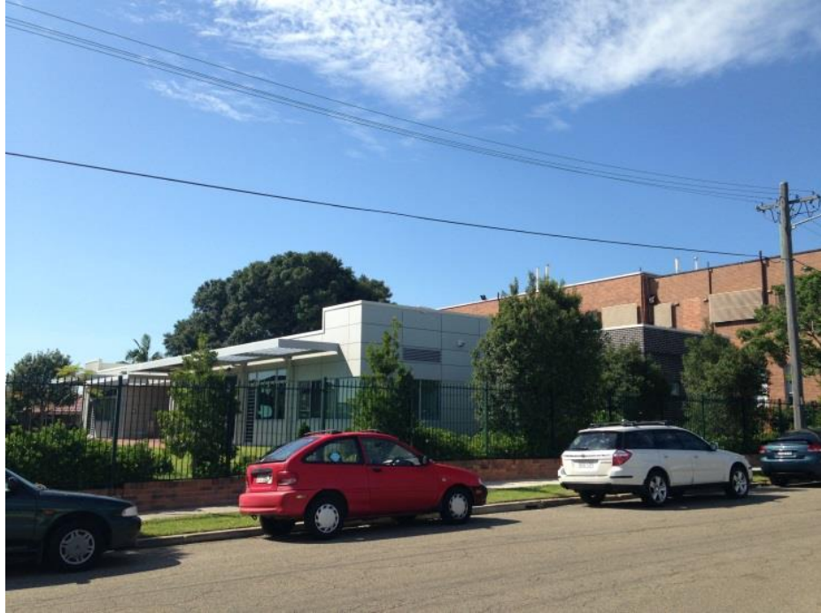
Figure 10 – Year Six Building on Grantham Street Source: JBA
