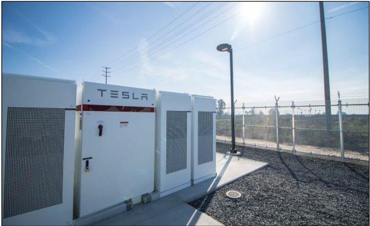
Figure 3-4: Typical BESS
