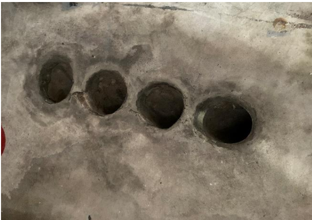
Photograph 9: Interior, substation floor, conduit penetrations following removal of asbestos-containing NC compound/caulking.
