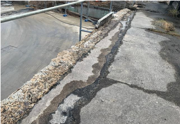
Photograph 3: Exterior, upper roof, following removal of remnant asbestos-containing white/beige caulking to louvres.
