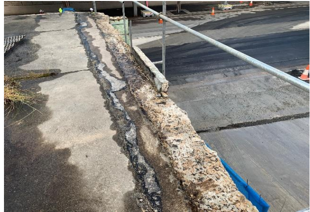
Photograph 4: Exterior, upper roof, following removal of remnant asbestos-containing white/beige caulking to louvres.
