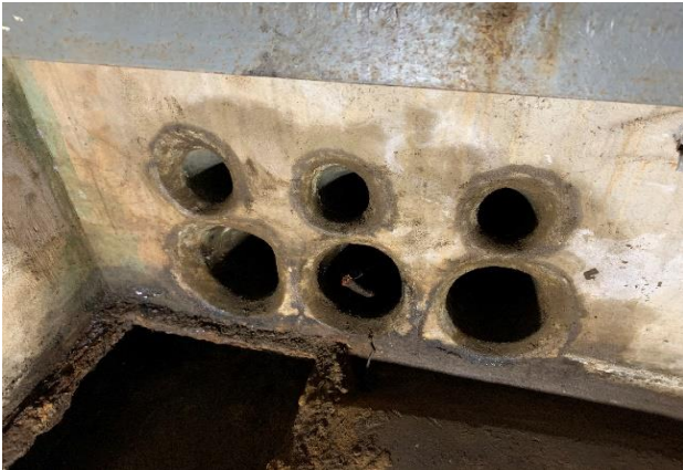
Photograph 9: Interior, substation floor, conduit penetrations following removal of asbestos-containing NC compound/caulking.
