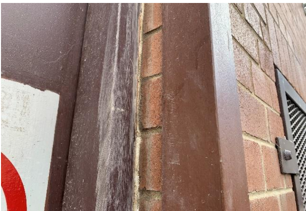
Photograph 5: Exterior, doorway following removal of asbestos-containing caulking.
