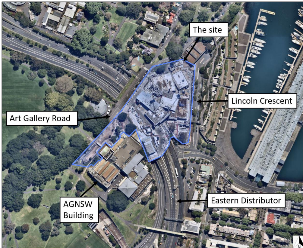
Figure 2 | Aerial view of the site looking north (Base source: Nearmap)
