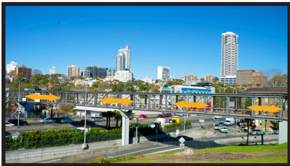
fig.01: Public Access Maintained
