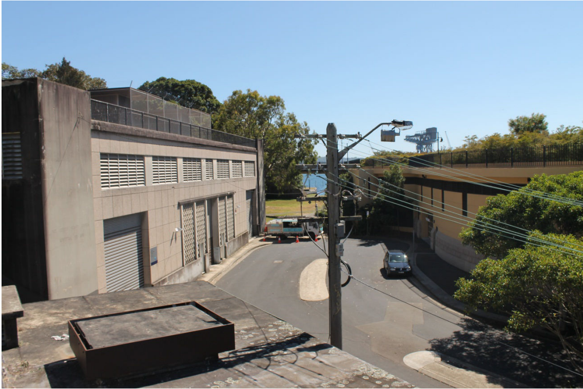
Figure 9 – Neighbouring Ausgrid substation on Lincoln Crescent
