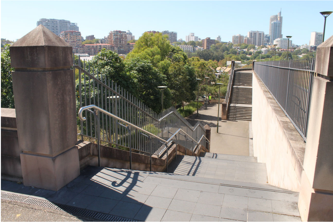
Figure 11 – Stairs leading up to northern side of land bridge
