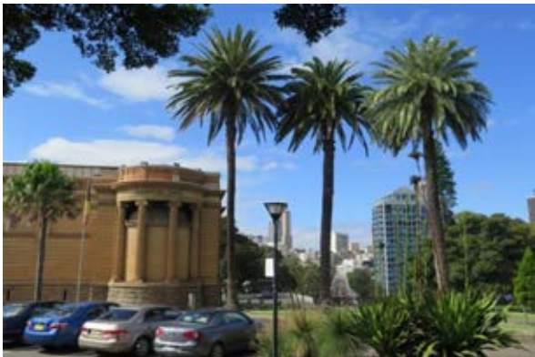
Figure 3.3 Engaged half-domed stair drum at the southern pavilion, accentuated by a ionic colonnade. (Source: GML Heritage, March 2016)
