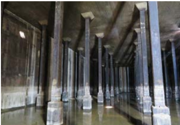
Figure 3.36 Interior of the Oil Tanks showing the column details and general spacing. (Source: GML Heritage 2017)
