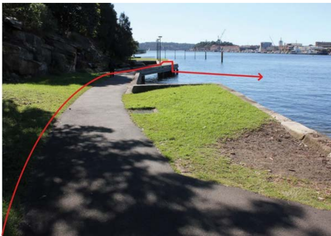
Figure 6.8 Photograph of the Woolloomooloo foreshore, looking north, showing the proposed route of the seawater heat exchange pipework along the foreshore and suspension under the timber walkway. (Source: GML 2016)
