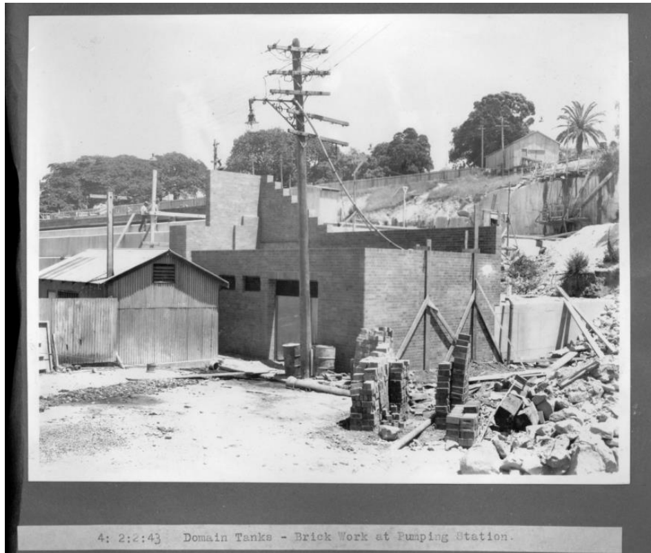
Figure 2.24 Pumping station under construction, dated 1943. (Source: Sydney Water Archives)
