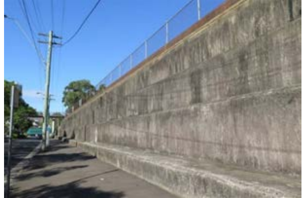
Figure 3.35 The stepped retaining wall along Lincoln Crescent which defines the tank's boundary on the eastern side. (Source: GML Heritage, 2016)
