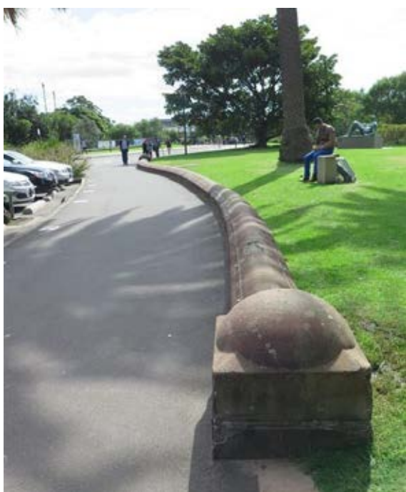
Figure 3.5 Low stone wall with semi-spherical capping stone detail, which defined the original semicircular carriageway at the front of the primary carriageway. (Source: GML Heritage, March 2016)
