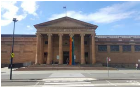
Figure 3.1 Front façade of the Art Gallery of NSW, showing four completed bas-reliefs filling the blind windows to the south of the portico. The lanterns installed over the vaulted skylights of the Grand Courts are visible above the parapet line. (Source: GML Heritage, March 2016)
