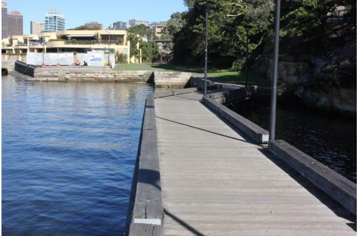
Figure 5.29 Photograph of the timber walkway along the Woolloomooloo foreshore, looking south towards Lincoln Crescent. (Source: GML 2016)
