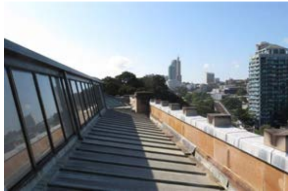
Figure 3.14 Exterior view of the artificial lantern system set over the court skylights. (Source: GML Heritage, March 2016)
