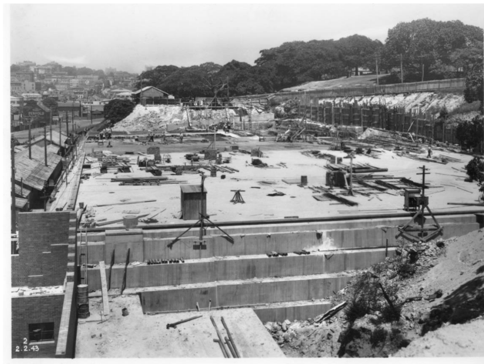
Figure 2.23 View south across the construction site, showing the stepped northern retaining wall and the lower concrete roof of the pump room in the foreground, taken February 1943. (Source: Sydney Water)
