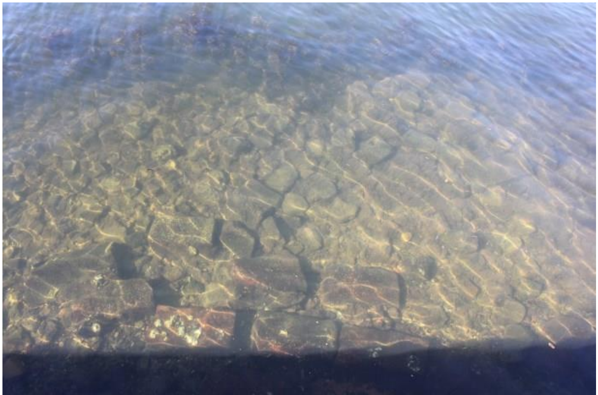
Figure 5.30 Example of the dressed and broken sandstone masonry underwater at the location of Robinson's Ladies Baths. (Source: GML 2016)
