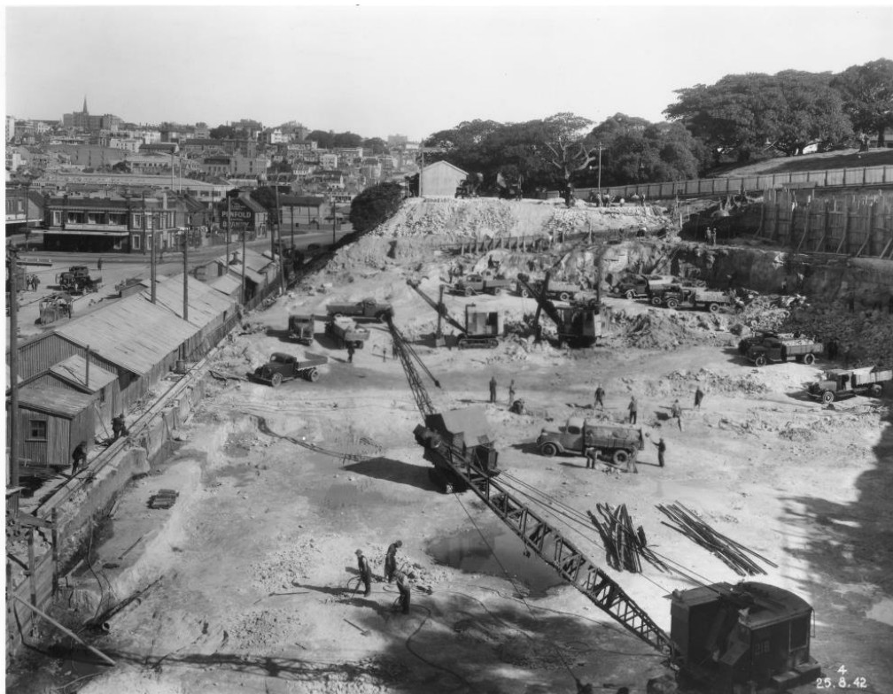
Figure 5.16 Excavation for the Domain Oil Tanks looking south, dated August 1942. (Source: Sydney Water Archives)
