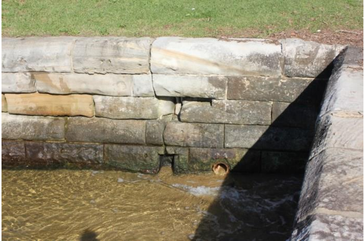
Figure 5.33 Example of existing outlets through the sandstone seawall. (Source: GML 2016)
