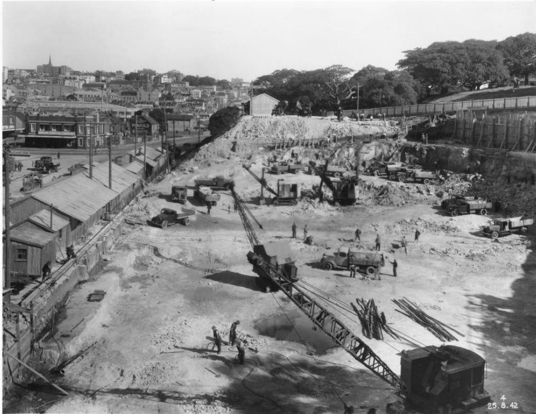
Figure 2.20 Excavation for the Domain Oil Tanks looking south, dated August 1942. (Source: Sydney Water Archives)
