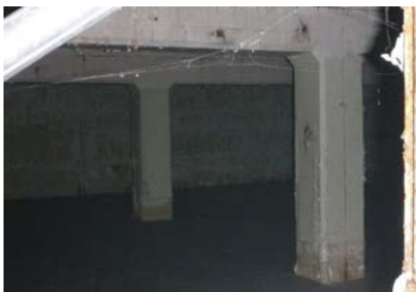
Figure 3.40 The reinforced concrete columns and beams of the pump room. (Source: GML Heritage, 2014)
