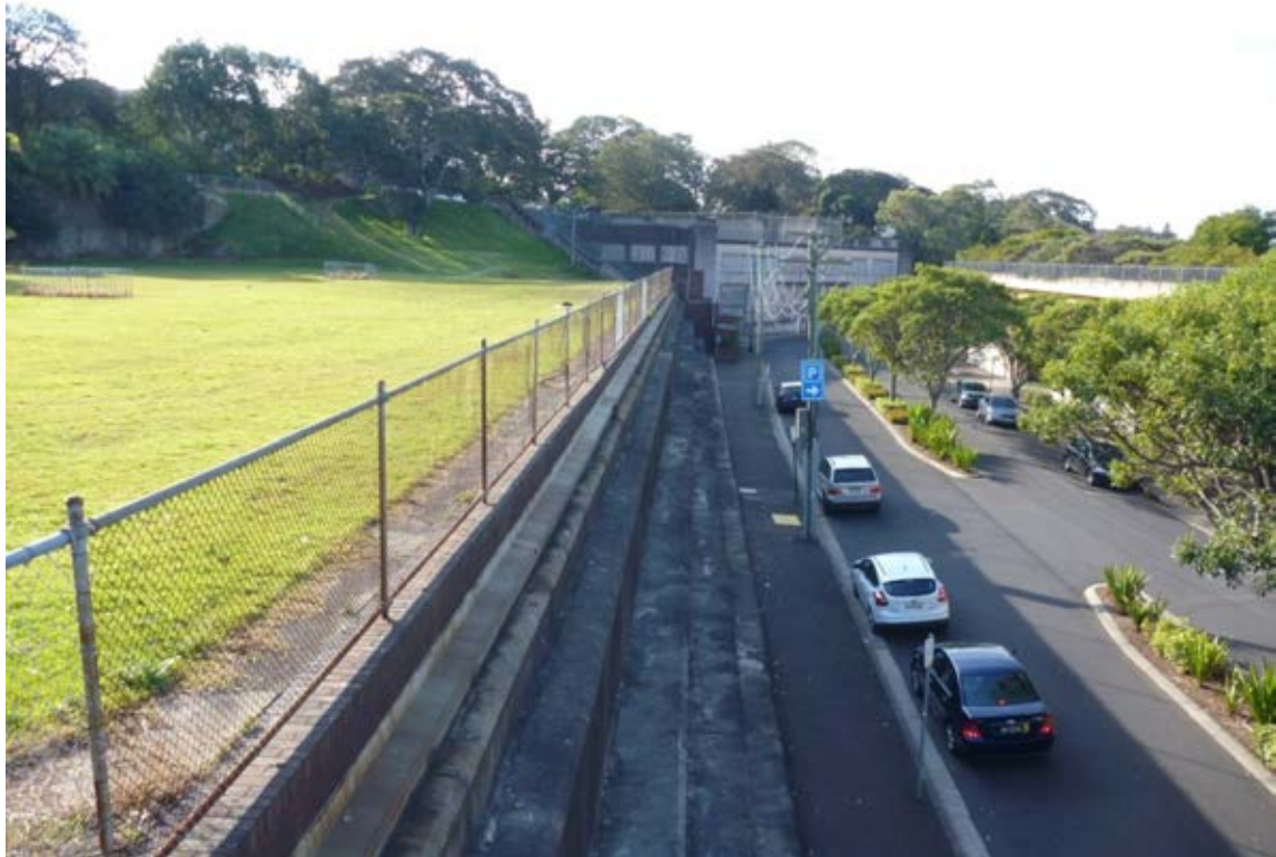
Figure 5.21 View of the Domain Oil Tanks from the pedestrian bridge over Lincoln Crescent. The stepped retaining wall is at the centre of the image, with the roof of the tanks on the left. (Source: GML 2014)
