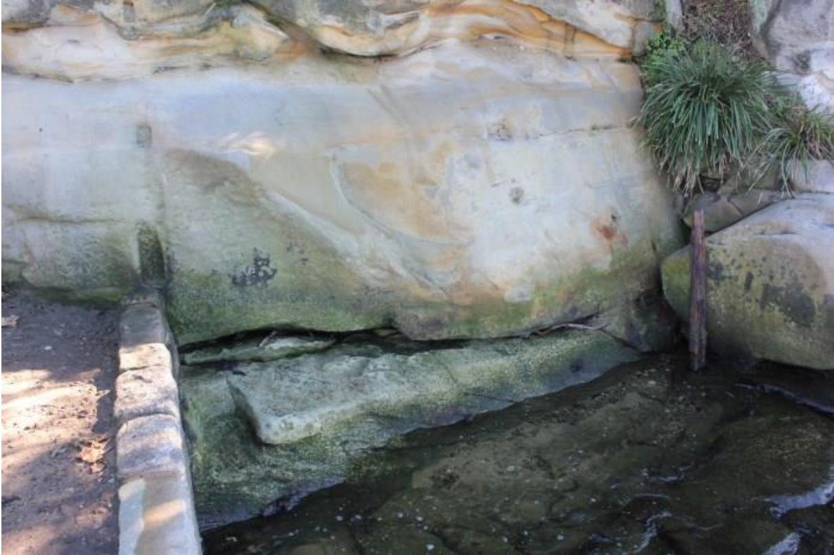
Figure 5.31 Photograph of remnants of the Robinson's Ladies Baths and modifications to the sandstone wall. (Source: GML 2016)
