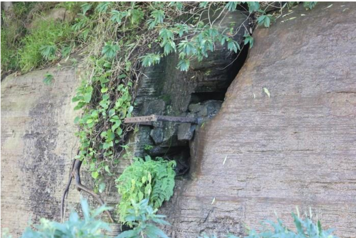
Figure 5.32 Detail of one of the modifications to the Domain sandstone walls. (Source: GML 2016)
