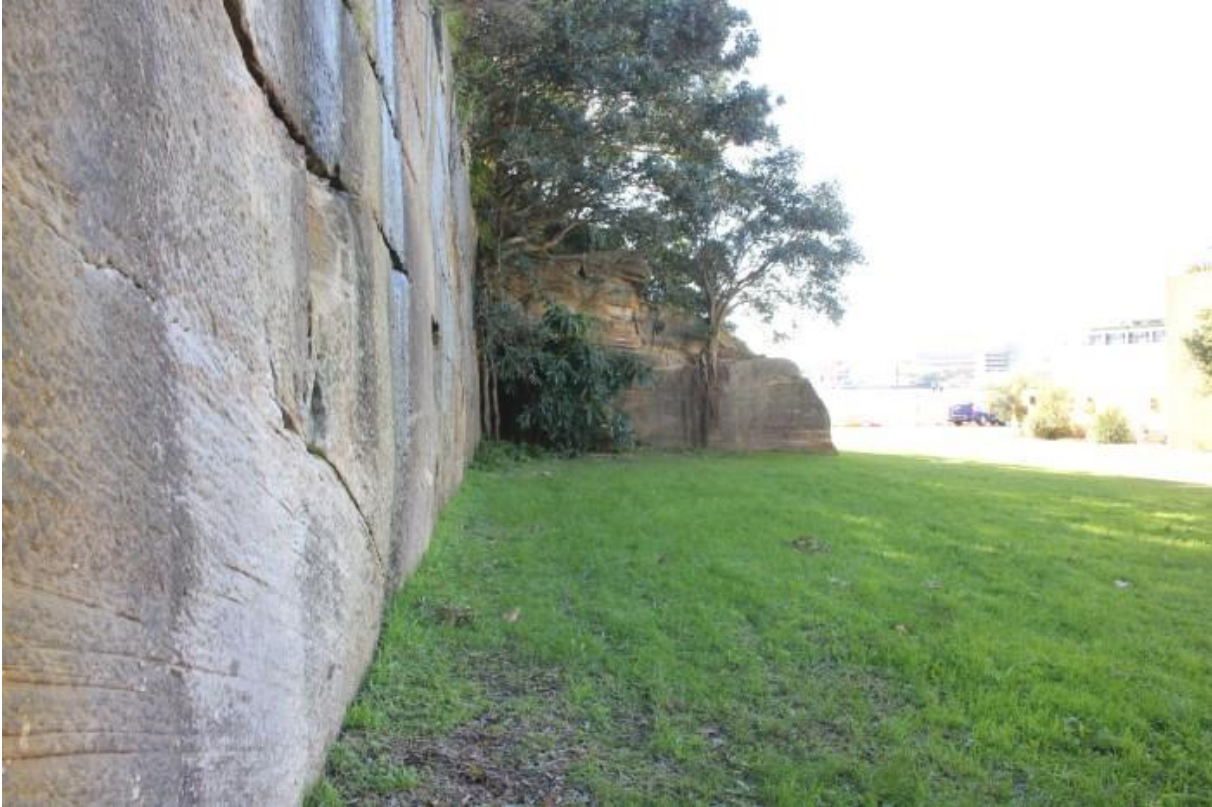
Figure 5.27 Photograph of the cut sandstone cliff faces along the Woolloomooloo foreshore. (Source: GML 2016)
