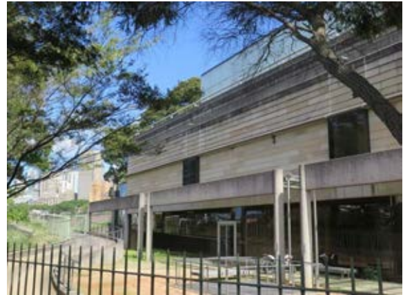
Figure 3.10 Continuation of sandstone veneer panelling along the exterior of the Bicentennial Wing, above which a terraced area sits surrounded by a steel railing. (Source: GML Heritage, March 2016)
