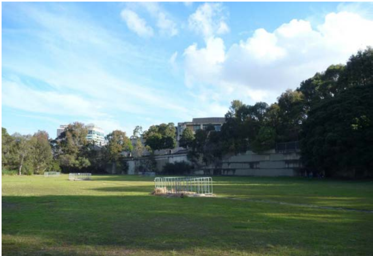
Figure 5.22 View south across the turfed roof of the tanks toward the Gallery. The stepped retaining wall along part of the rear of the tanks is shown in the centre of the image. (Source: GML 2014)
