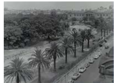
Figure 2.30 Macquarie Street, Sydney, 1959. Site works for the Eastern Distributor, showing trees in the Royal Botanic Gardens. (Source: City of Sydney Archives, File 010/010881, NSCA CRS 48/881)
