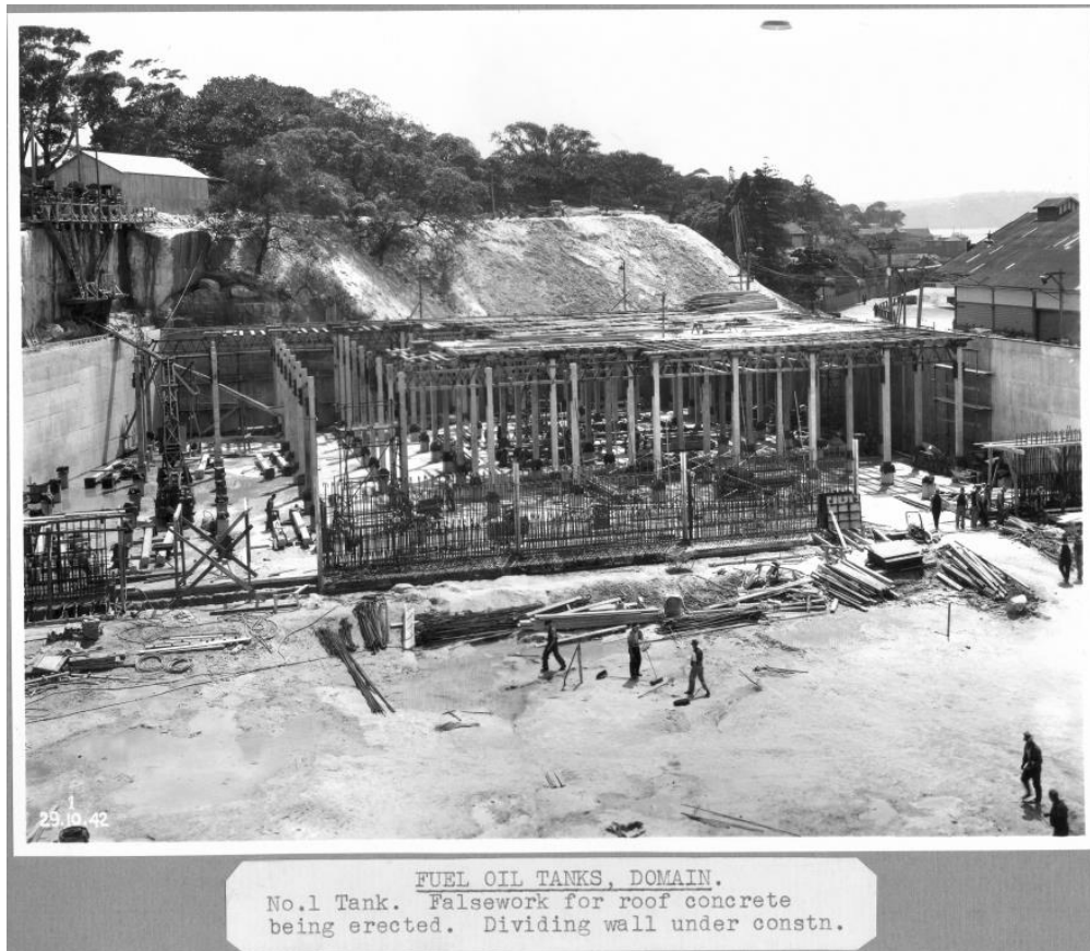
Figure 2.22 Concrete columns in place for the northern tank and timber formwork being laid to support the concrete roof. The dividing wall between the two tanks is shown under construction, taken October 1942. (Source: Naval Historical Society)
