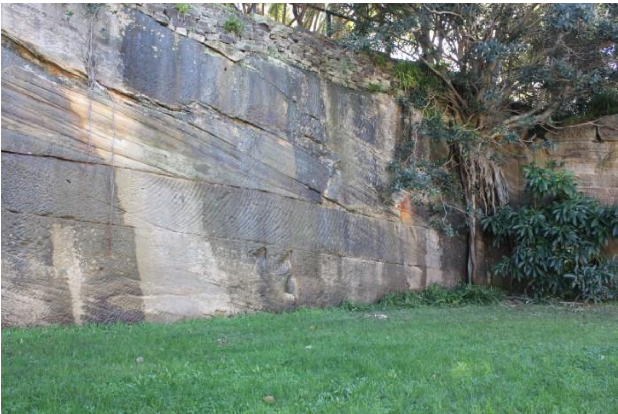
Figure 5.28 Photograph of the cut sandstone faces along the Woolloomooloo foreshore, showing evidence of the use of a circular rock saw. (Source: GML 2016)
