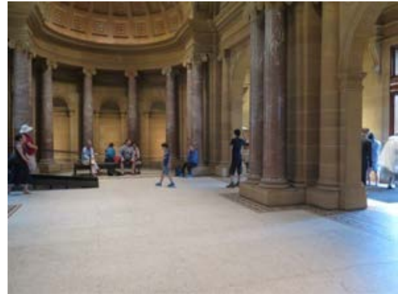
Figure 3.16 The oval-shaped entrance vestibule with mosaic tile floor, Ionic columns fashioned from Kempsey marble, and walls and ceilings of Maroubra sandstone. (Source: GML Heritage, March 2016)
