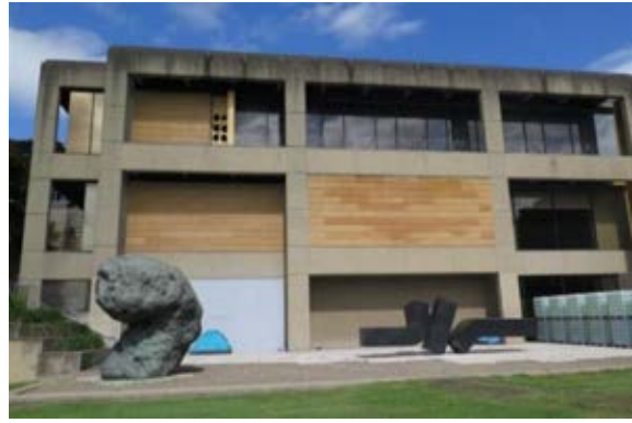
Figure 3.8 Northeast elevation, predominated by the Captain Cook Wing. Large-scale, free-standing sculptures curated by the Gallery help to emphasize the brutalist undertones of the architecture and expand the curtilage of the building. (Source: GML Heritage, March 2016)
