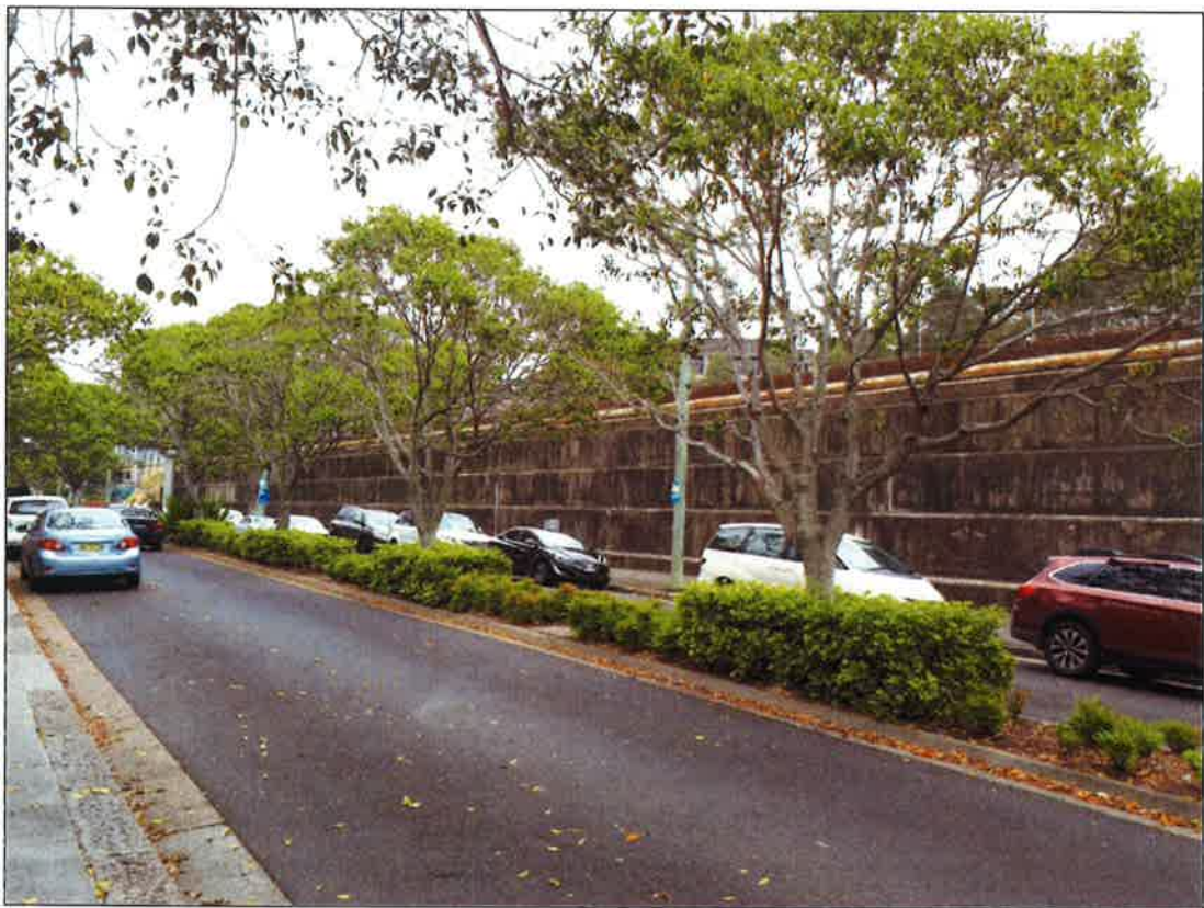
Figure 51 | Fuel bunker eastern wall viewed from Lincoln Crescent (Source: Department's photograph)
