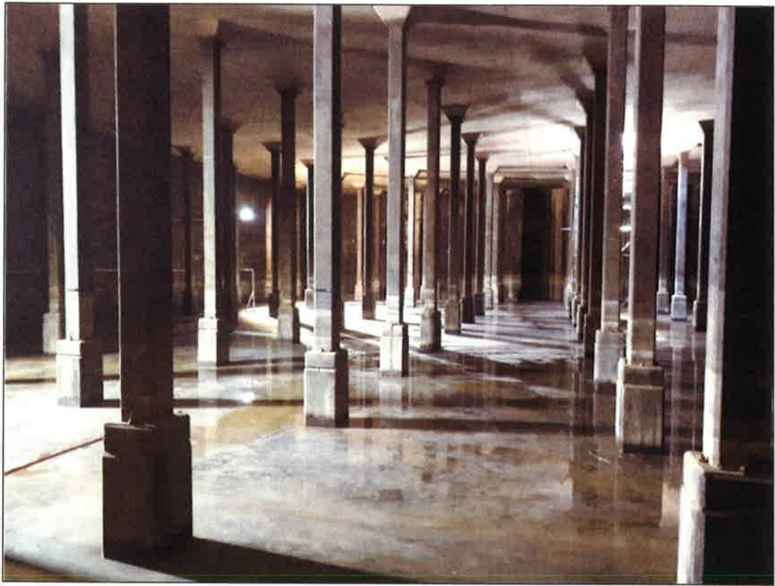
Figure 50 | The southern fuel bunker (Source: Department's photograph)
