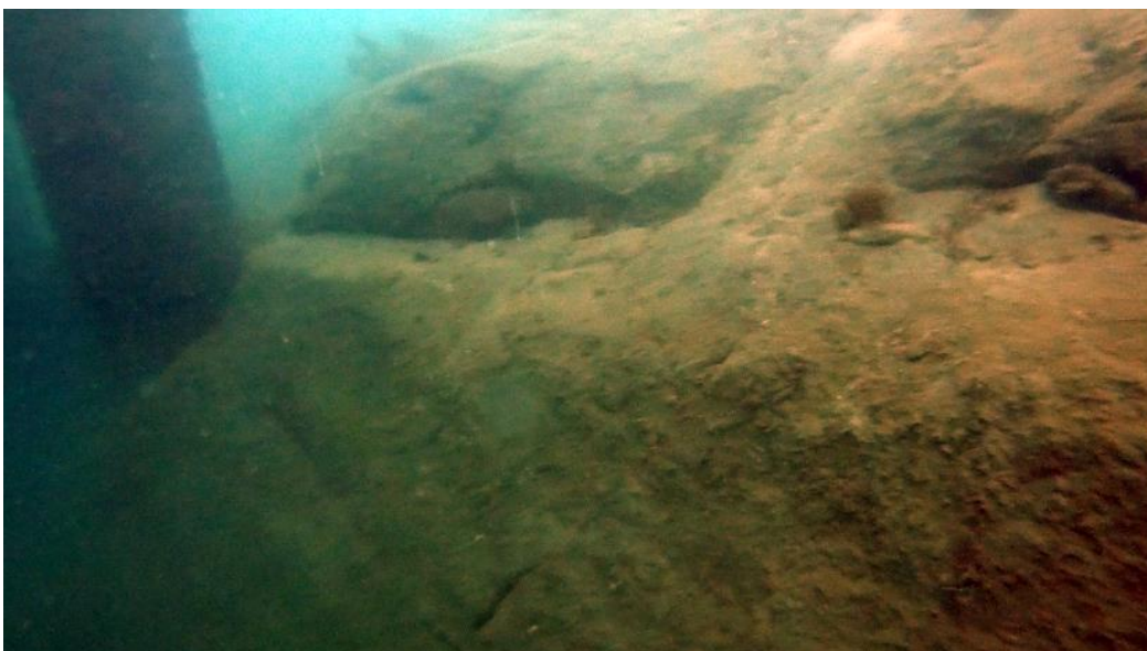
Photograph 6: Target 7, natural rock adjacent to pile associated with marina berth
