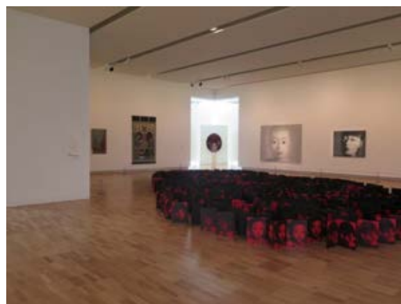
Figure 3.28 The upper Asian Gallery at ground level, showing a modern ceiling concealing services and blue gum flooring. (Source: GML Heritage, March 2016)
