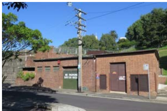
Figure 3.38 The single-storey brick pump house from the Lincoln Crescent frontage. (Source: GML Heritage, 2016)
