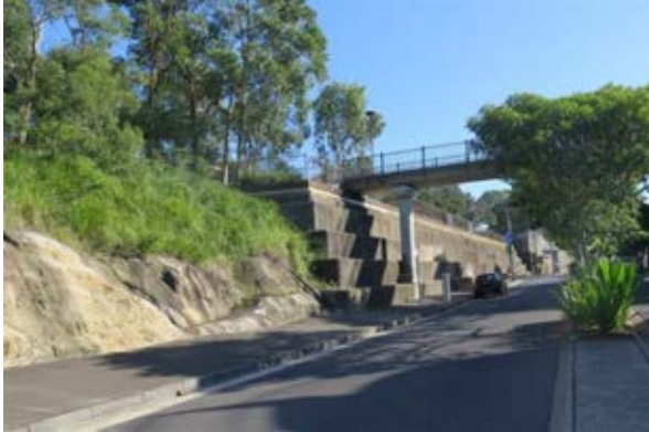
Figure 3.34 The dominated form of the concrete stepped retaining wall, looking north along Lincoln Crescent. (Source: GML Heritage, 2016)
