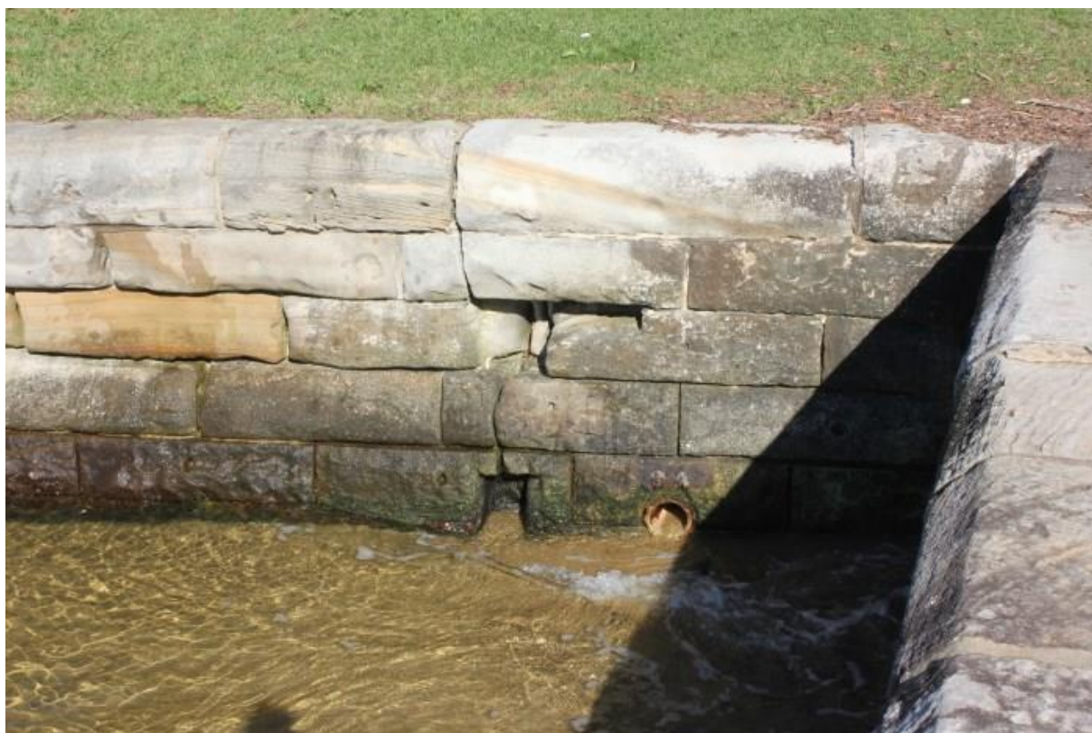
Figure 5.31 Example of existing outlets through the sandstone seawall. (Source: GML 2016)
