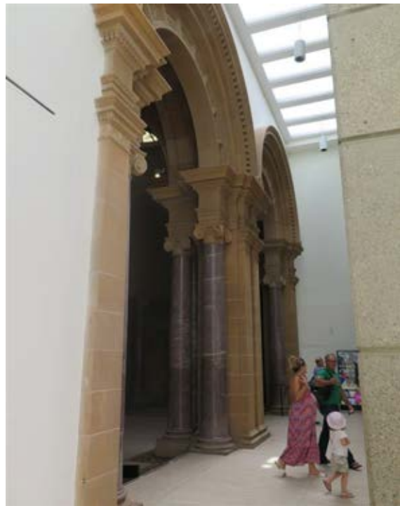
Figure 3.20 Juncture between the Vernon vestibule and the Captain Cook addition, showing the treatment of the arched entranceway via a void space lit with natural light from above. (Source: GML Heritage, March 2016)
