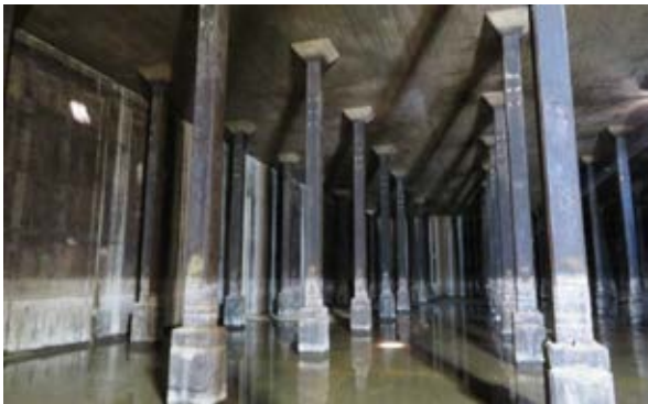
Figure 3.36 Interior of the Oil Tanks showing the column details and general spacing. (Source: GML Heritage 2017)
