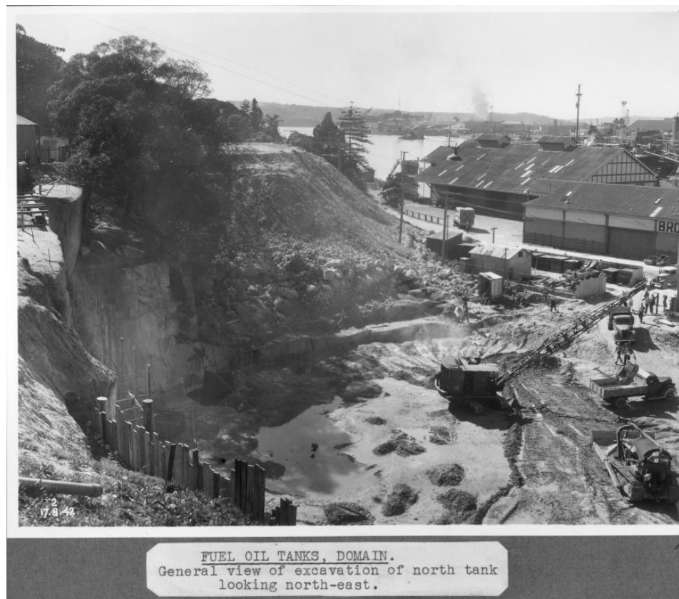
Figure 2.19 Excavation for the Domain fuel tanks, dated August 1942. (Source: Naval Historical Society)
