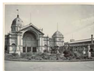
Figure 2.5 Royal Exhibition Building, Melbourne, 1885–1890. (Source: State Library of Victoria, H84.202/20)
