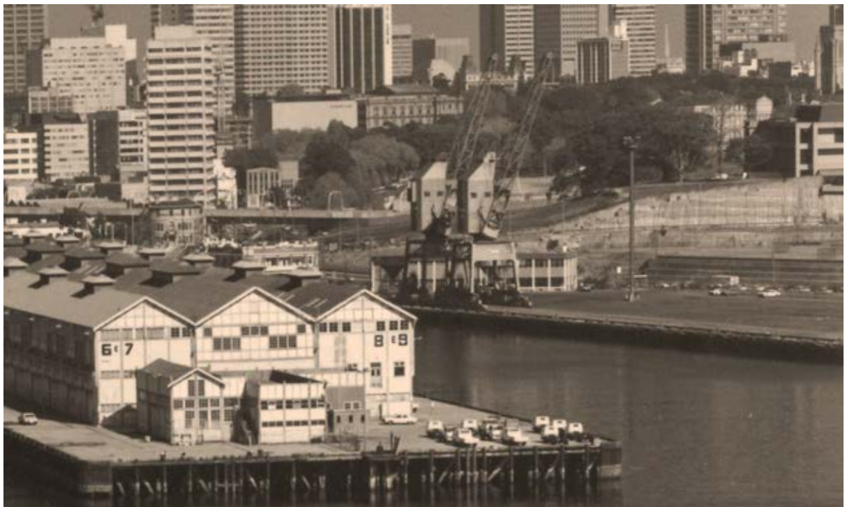
Figure 2.25 A c1980s view looking southwest across Woolloomooloo Bay to the site of the oil tanks. The stepped concrete retaining wall in front of the tanks is shown fronting Lincoln Crescent. Note the apartments on Woolloomooloo Bay have not yet been constructed. (Source: Naval Historical Society)
