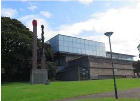
Figure 3.9 The stepped rear elevation of the Art Gallery of NSW, with the 2003 Asian Galleries sitting atop the Bicentennial Wing structure. (Source: GML Heritage, March 2016)
