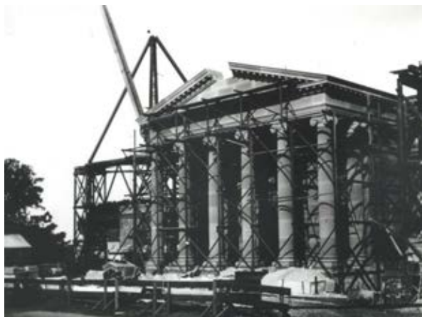
Figure 2.34 Portico under construction, completed in 1902. (Source: Art Gallery of NSW)
