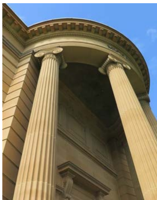
Figure 3.6 Articulated end pavilion at the northwestern corner of the Vernon building, with Ionic columns, dentil moulding to the cornices, and frieze above with brass lettering. (Source: GML Heritage, March 2016)
