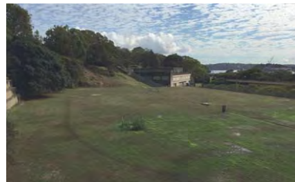
View of existing fuel bunker roof surface, taken from the southern access path facing north east towards Garden Island. Source: Architectus, 6 February 2018
