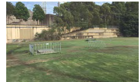
View of existing fuel bunker roof surface, access hatches retaining structures and the Eastern Distributor land bridge and taken from the eastern perimeter of the roof surface facing west towards the city. Source: Architectus, 6 February 2018
