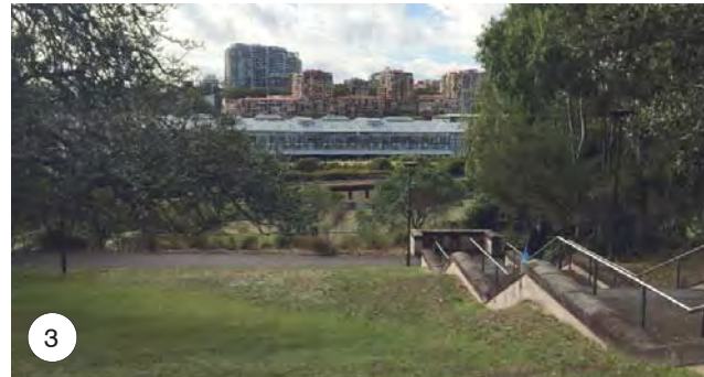
View from staircase facing site
