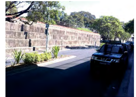
Photo of fuel bunker steps at Lincoln Crescent Source: Architectus
