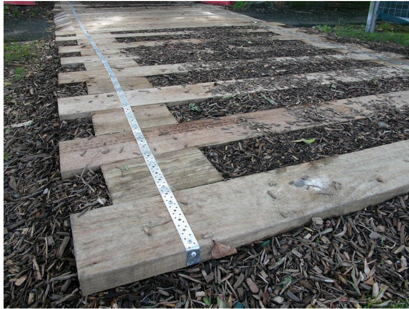
Figure 5 – Showing typical detail for rumble boards.
