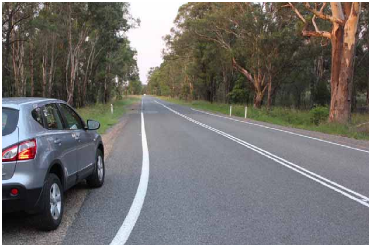
Photograph 2.8 Broke Road/MTO CHPP access intersection looking north
