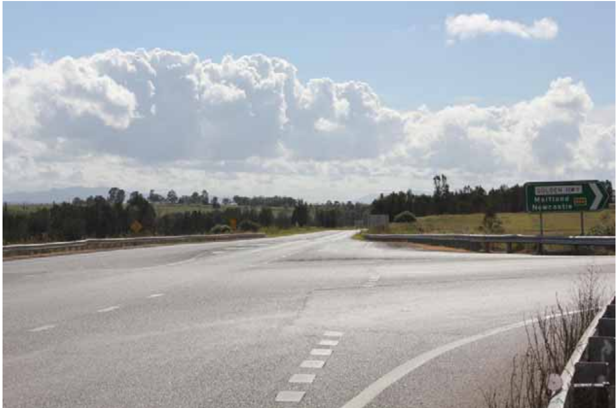
Photograph 2.1 Golden Highway/Mitchell Line Road intersection looking east
