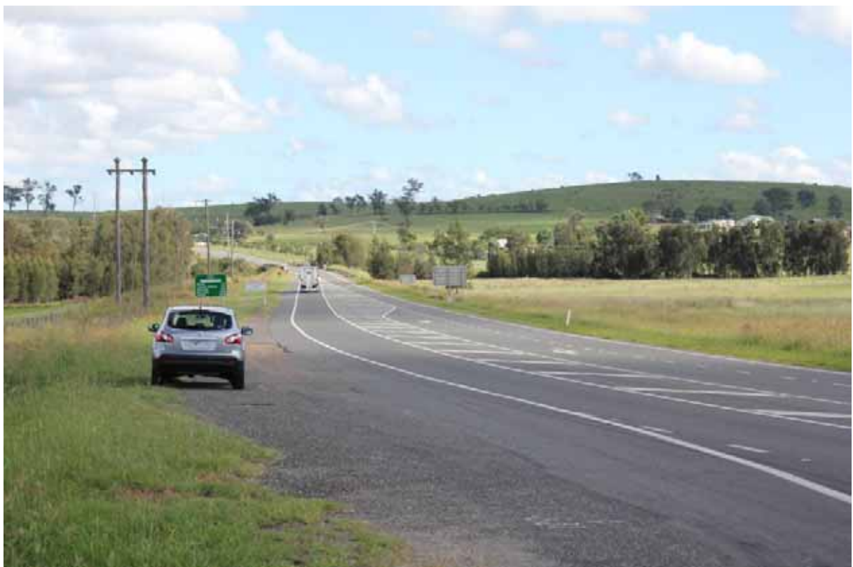
Photograph 2.4 Golden Highway/Broke Road intersection looking west
