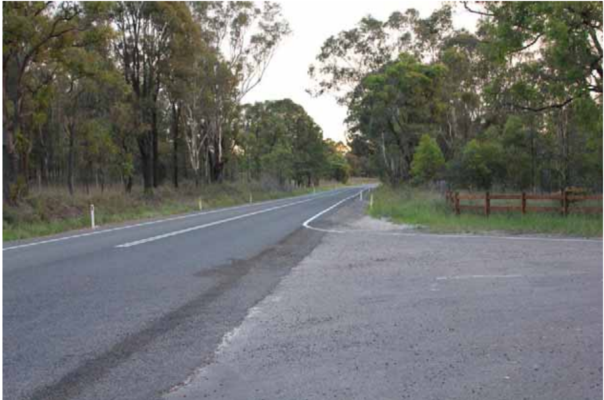
Photograph 2.7 Broke Road/MTO CHPP access intersection looking south
