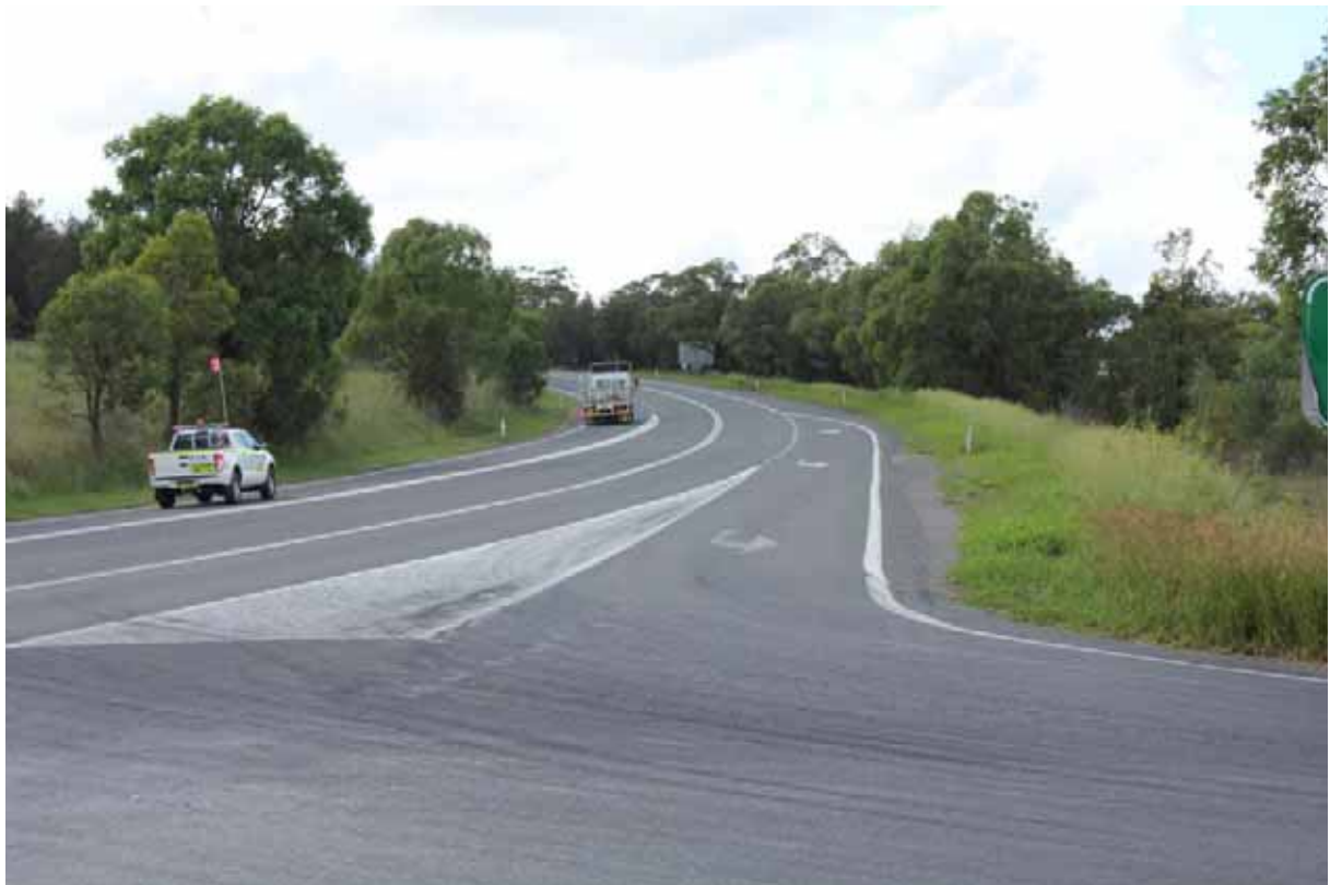
Photograph 2.3 Golden Highway/Broke Road intersection looking east
