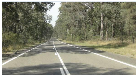
Putty Road looking west
