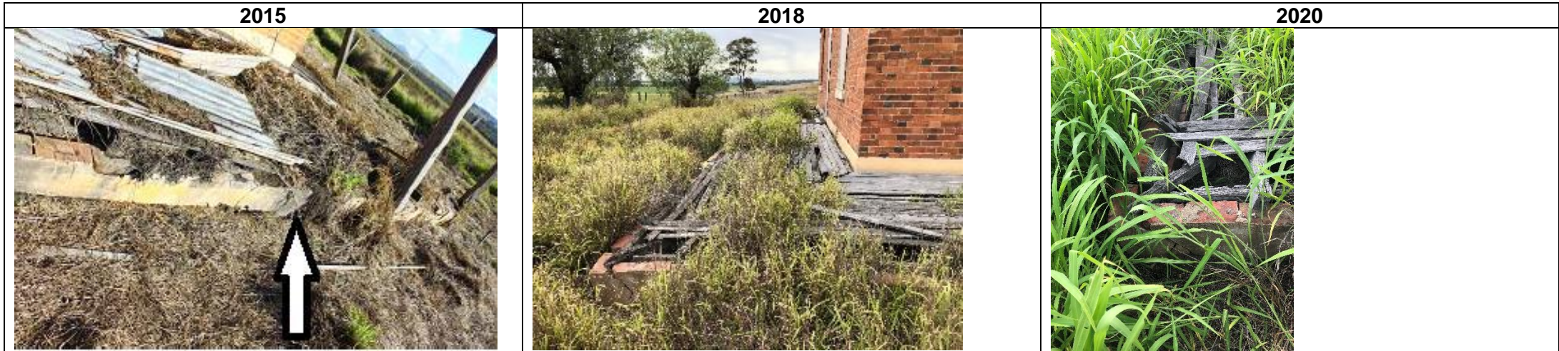
View of eastern verandah (focus on dwarf wall)
