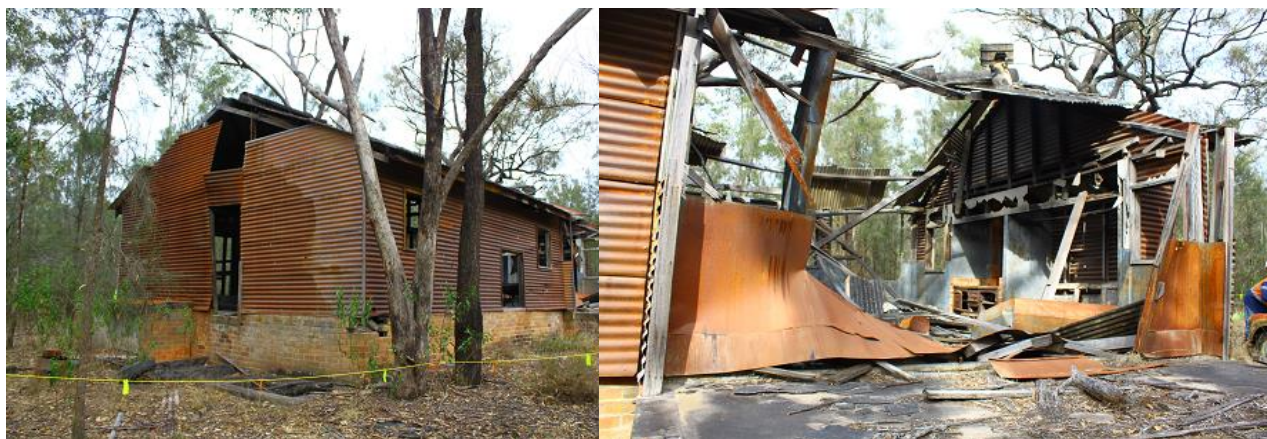
View to mess from south-east (2012)
