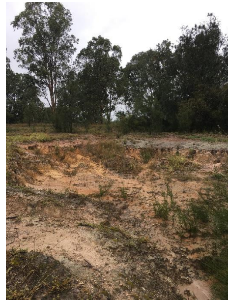
Plate 37 Erosion (top of right bank)
