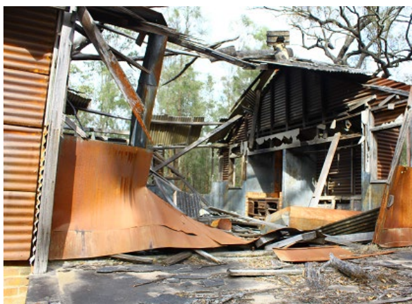
Remnant kitchen area (2012)
