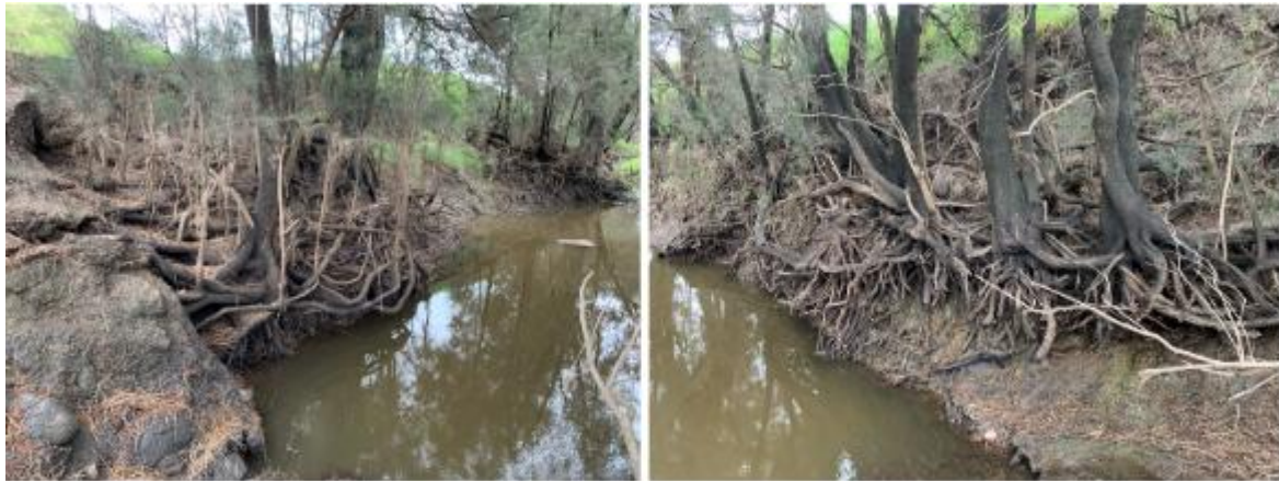
Figure 42: LC10 left bank (left) and right bank (right).
