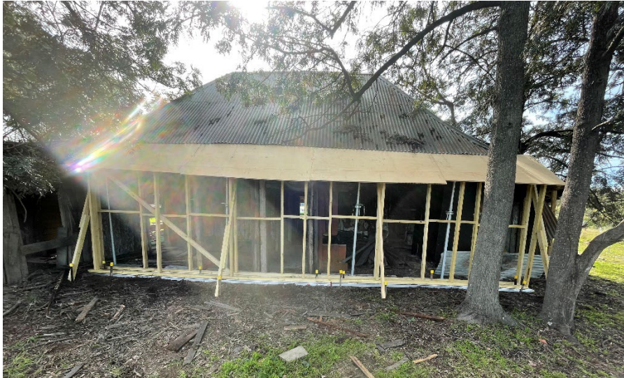
FIGURE 24: TEMPORARY ROOFING EXTENSION AND SUPPORTING FRAMEWORK AT REAR OF SPRINGWOOD HOMESTEAD
