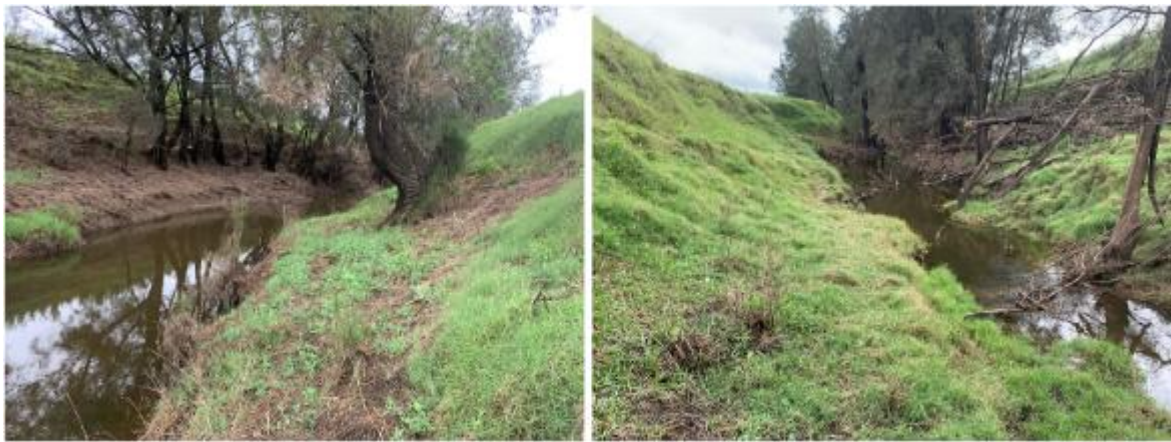
Figure 43: Site LC15 looking upstream (left) and looking downstream (right).
