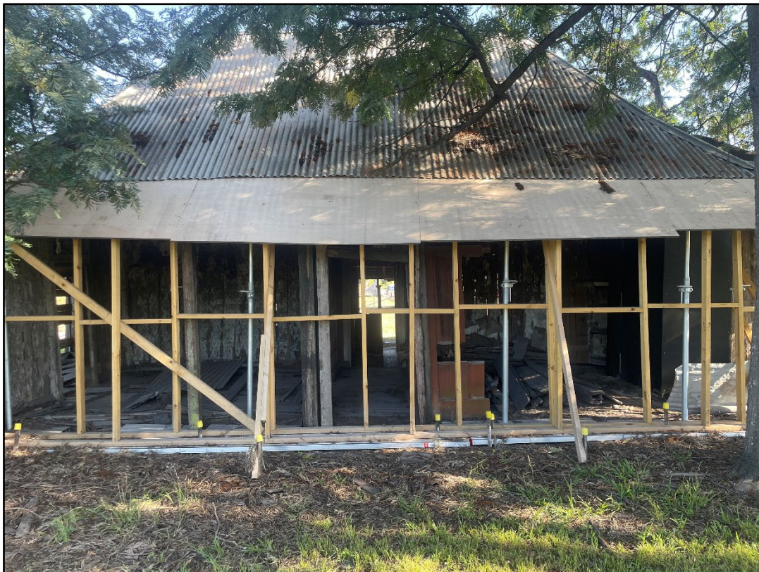
Recent temporary roof extension and supporting framework installed along southern elevation within the last 12 months
