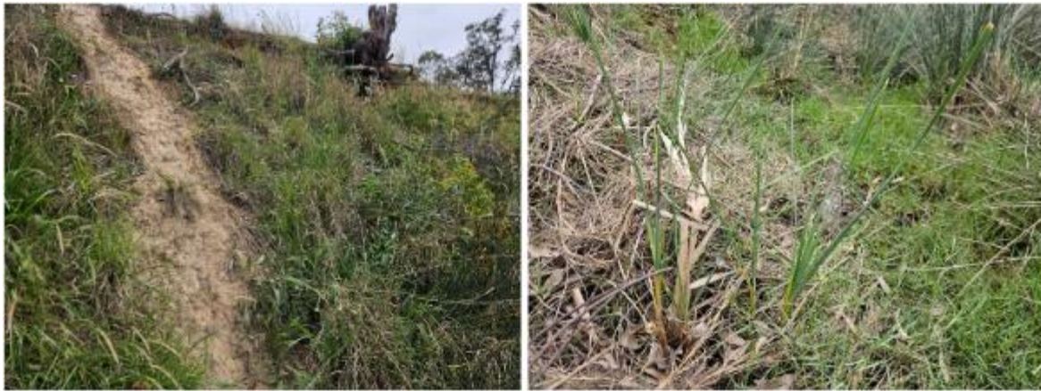
Figure 21: Animal tracks and active erosion blocked via felled trees.
