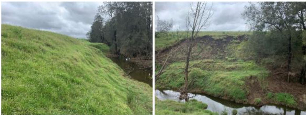
Figure 44: LC15 left bank (left) and right bank (right).
