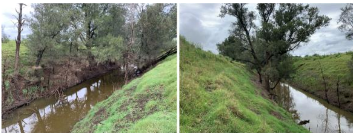
Figure 45: Looking upstream (left) and downstream (right) at LC13.
