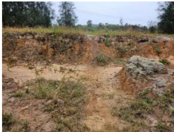
Figure 7: Erosion scar along the upper right-hand bank.
