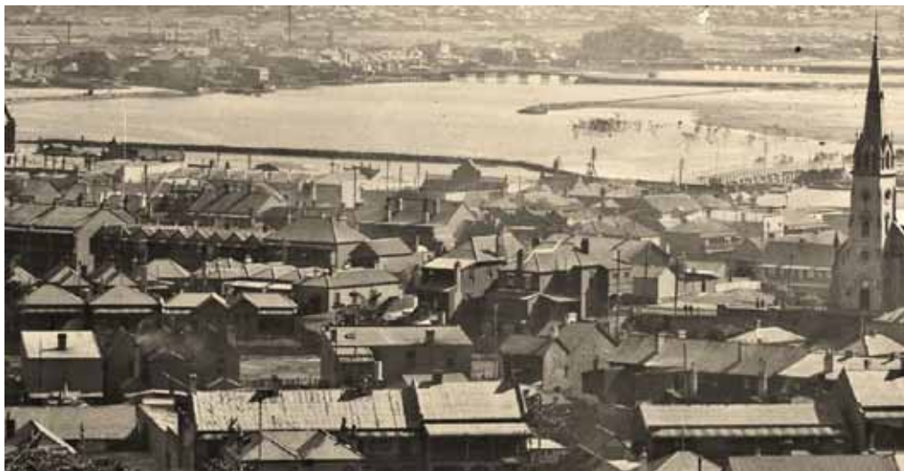
Figure 16. Figure 17. Detail of above view, showing Lucerna , Larken's weatherboard cottage and brick cottages, Hackworthy's Terrace and Devon Terrace. Davis' nine-dwelling terrace is to the left.
