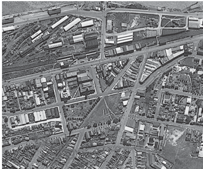
Figure 19. Figure 20. Figure 21. Aerial View, 1944. The location of Lucerna , Hackworthy's Terrace and cottages, Wascoe's cottage, Devon Terrace and Larken's cottages is shown. Newcastle City Council
