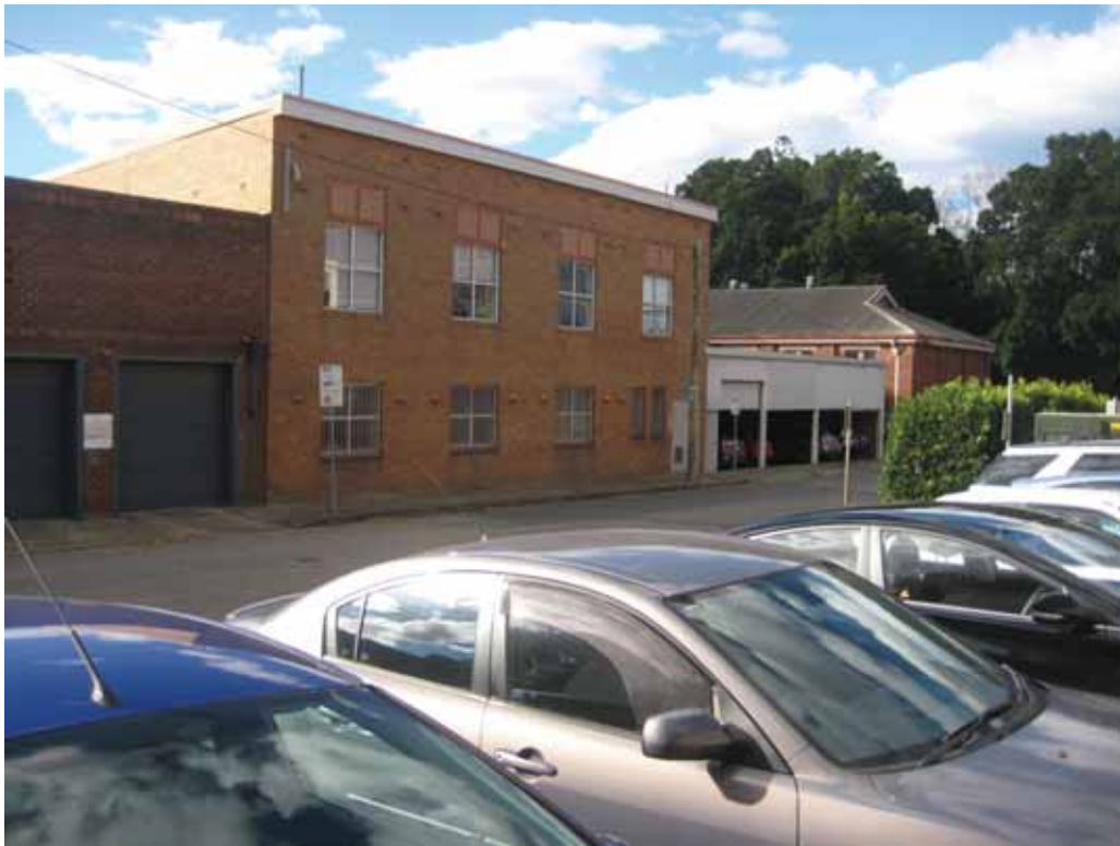
Figure 56. Looking north-east from existing Gibson Street car park to commercial development on opposite side of Gibson Street. The soon-to-be demolished Mackie's Building, partially obscured by the hedge, is at extreme right. EJE
