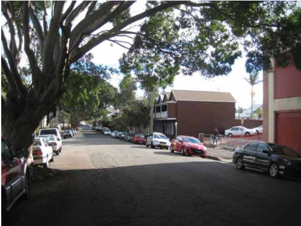
Figure 46. Looking north-west along Laman Street, showing Davis' Terrace, left, existing car park, middle, and Conservatorium, right. EJE
