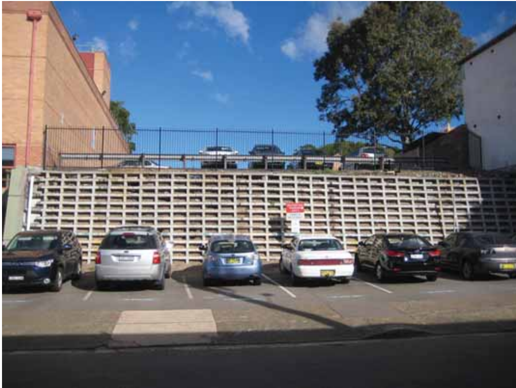
Figure 50. Closer view, looking south from Gibson Street. Note intrusive crib-lock retaining wall, and cars parked in car park addressing Laman Street. EJE
