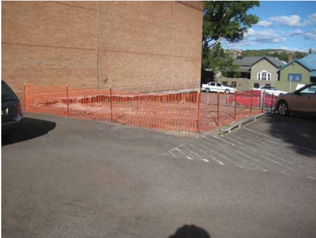
Figure 34. Existing car park, showing site of demolished cottage; Conservatorium is at left. EJE
