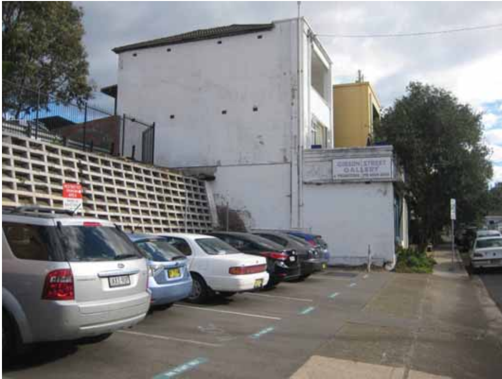
Figure 60. Relationship between existing Gibson Street car park and 15 Gibson Street (Gibson Street Gallery). EJE
