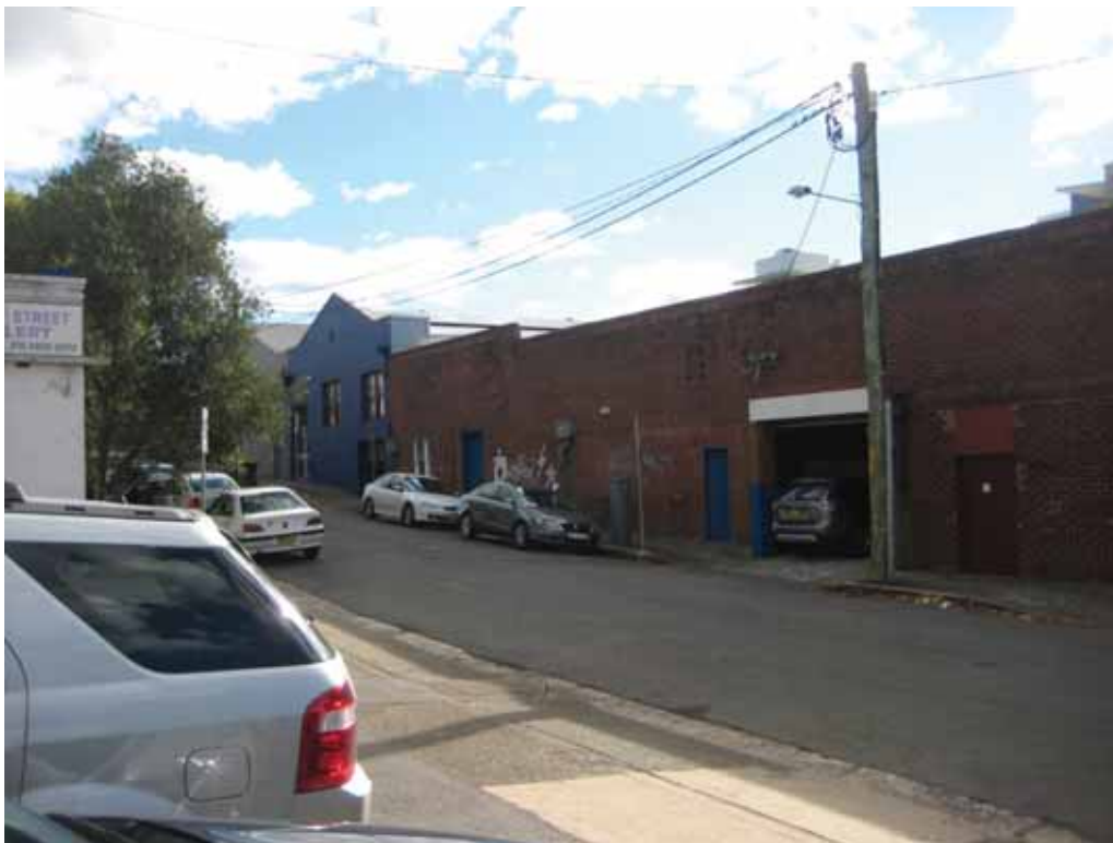
Figure 61. Commercial premises in Gibson Street; note roller doors, graffiti and generally nondescript appearance. EJE
