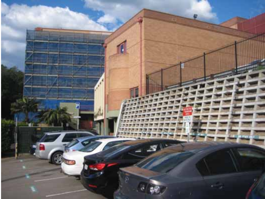
Figure 58. Existing Gibson Street car park, showing original (scaffolded) and 1988 Conservatorium buildings, with retaining wall at right. EJE
