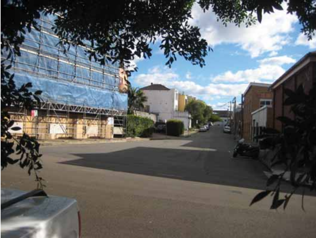
Figure 64. Looking west across Auckland Street from Civic Park footpath, showing existing Gibson Street car park and crib-lock retaining wall in middle distance. EJE
