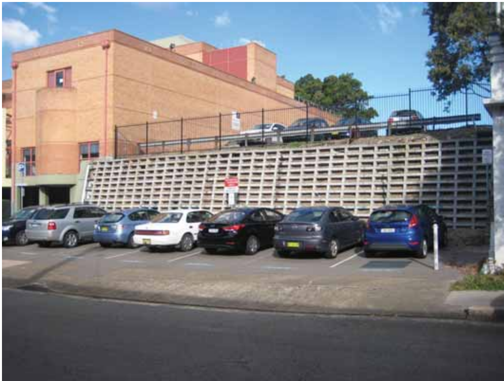
Figure 52. Existing Gibson Street car park, showing southern footpath of Gibson Street. EJE
