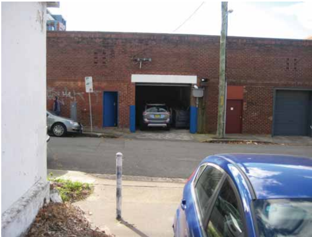
Figure 55. Looking north from car park to commercial development on opposite side of existing Gibson Street. Note roller doors. 15 Gibson Street (Gibson Street Gallery) is at left. EJE
