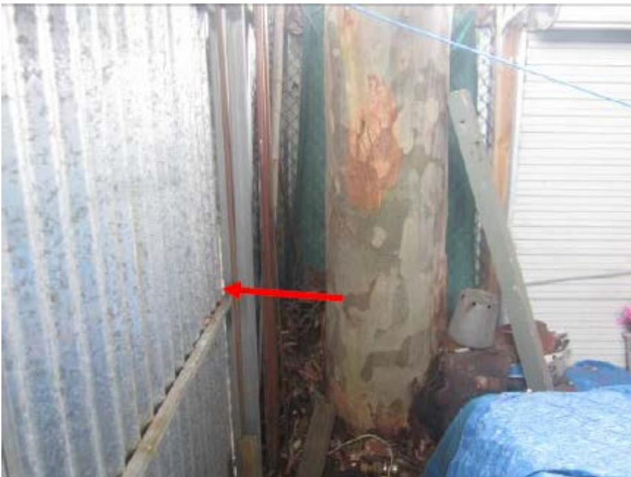
Figure 6 – Existing conditions of Tree 1
