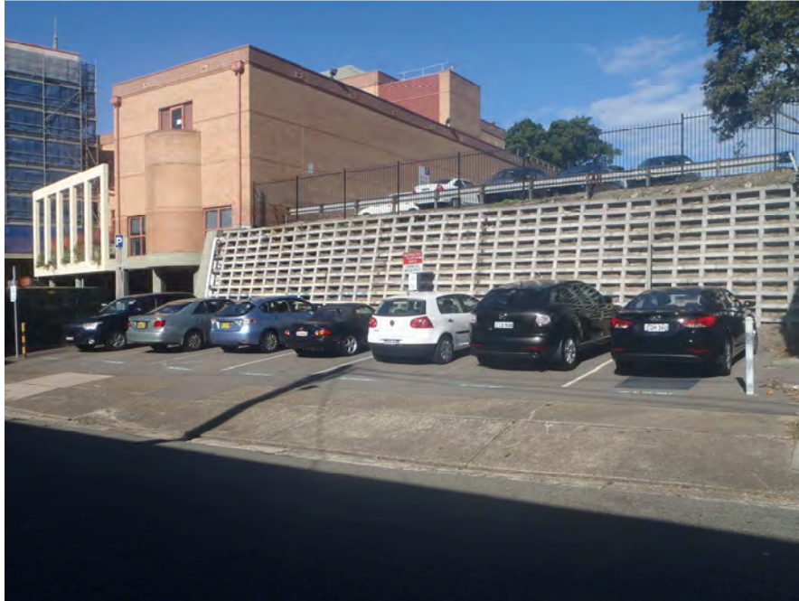
Figure 9 – Lower deck of the Laman Street Car Park Source: JBA
