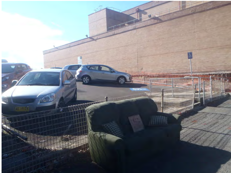
Figure 8 – Upper deck of the Laman Street Car Park Source: JBA
