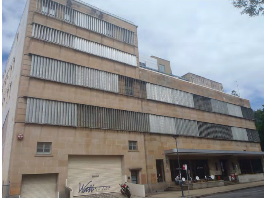
Figure 7 – View to NESCA House from Auckland Street Source: JBA
