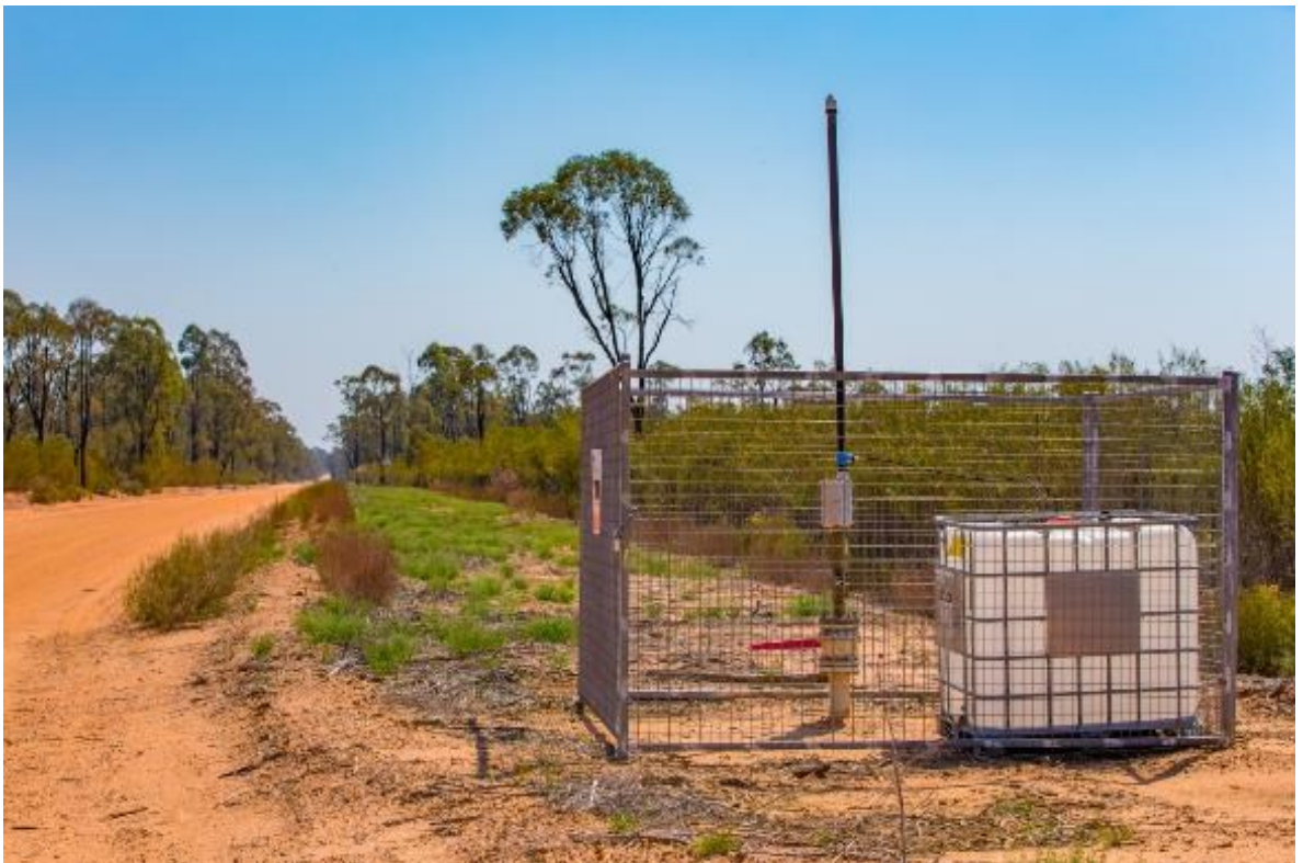
Figure 6-39 High point vent along gathering lines
