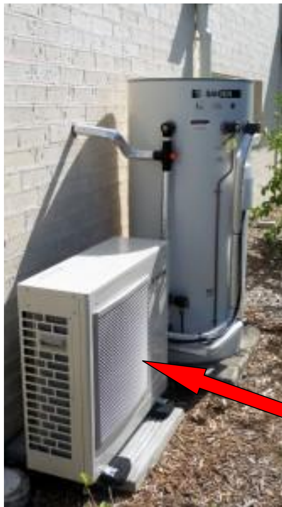
Figure 16: Heat-pump water heater (HPWH).
