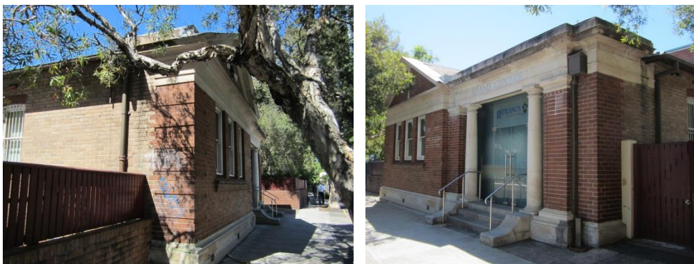
Figure 18 – Former Post Office now known as the Adams Centre, located on the southern side of Military Road, showing the North Elevation facing onto Military Road. Redlands, currently use Adams Centre as a dance studio (Source: NBRSPARTNERS, December 2013)
