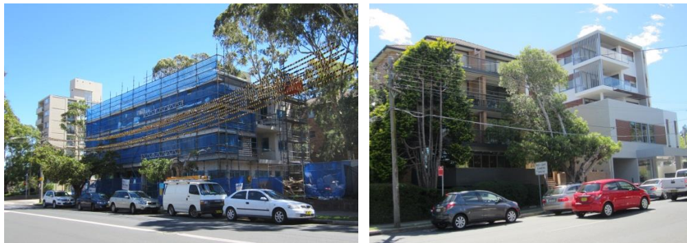
Figure 14 – View of Winnie Street showing medium residential development located on the eastern side of Winnie Street on the corner of Gerard Street (left) and Military Road (right) (Source: NBRSPARTNERS, December 2013)
