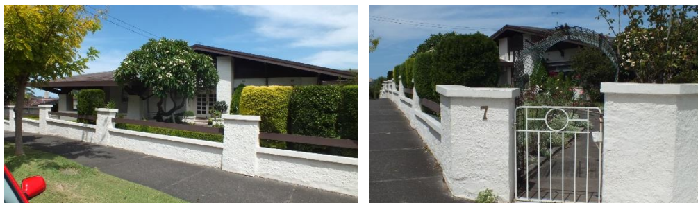
Figure 4 – View to “Belvedere”, 7 Cranbrook Avenue, Cremorne, identified as Heritage Item I0045. The heritage item is located on the corner of Cranbrook Avenue and Allister Street (Source: NBRSPARTNERS, February 2015)
