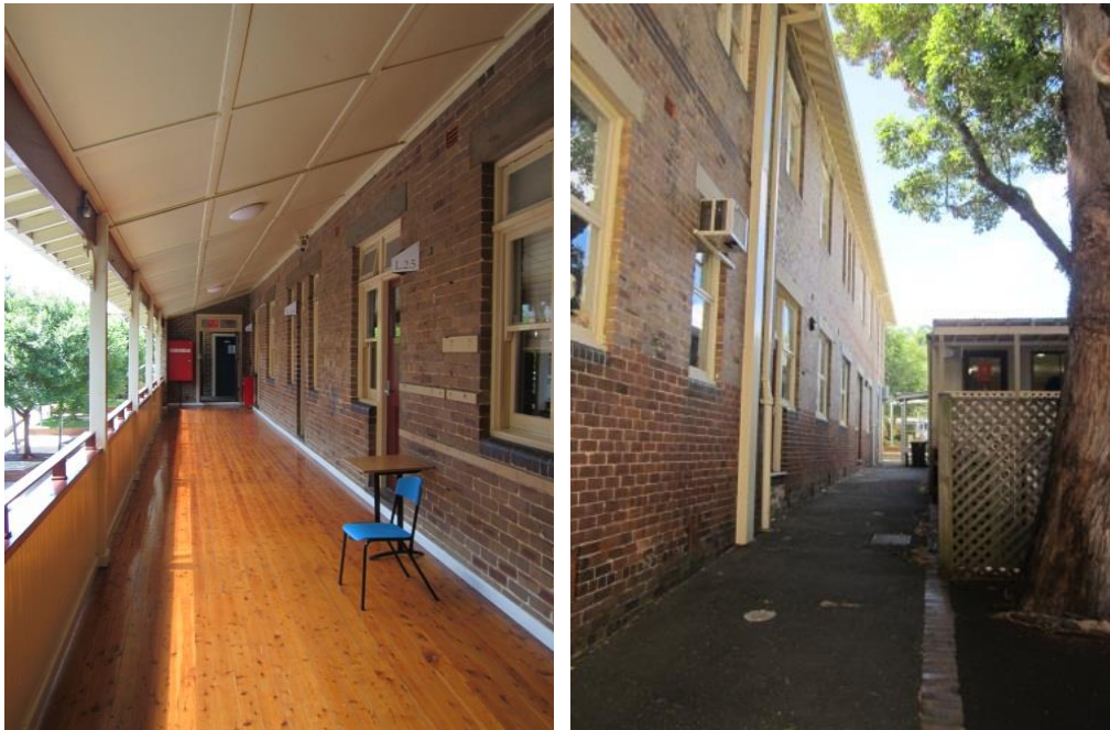
Figure 33 – Liggins Building, two-storey classroom block, showing first floor verandah leading to classrooms (left) and western elevation of the classroom block with demountable building adjoining to the west (Source: NBRSPARTNERS, December 2013)
