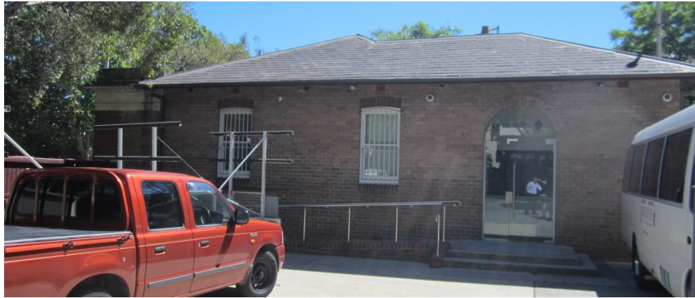
Figure 19 – Adams Centre, showing the West Elevation. The adjoining site is used as a parking area for Redlands vehicles (Source: NBRSPARTNERS, December 2013)
