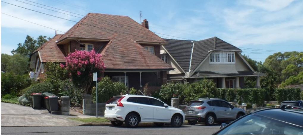
Figure 7 – View to Nos 32 and 34 Cranbrook Avenue, Cremorne, identified as Heritage Items of local significance on the North Sydney LEP. The two properties are located on the northern side of Cranbrook Avenue, opposite the State heritage listed items (Source: NBRS+PARTNERS, February 2015)
