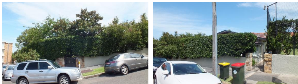
Figure 6 – View to “Esslemont”, 11 Cranbrook Avenue, Cremorne, identified as Heritage Item I0046. The heritage item is located east and downhill from the corner of Cranbrook Avenue and Allister Street (Source: NBRSPARTNERS, February 2015)
