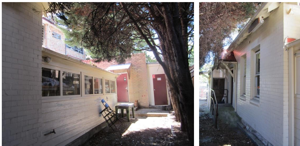
Figure 35 – A number of narrow circulation spaces are located between the learning spaces (Source: NBRSPARTNERS, December 2013)
