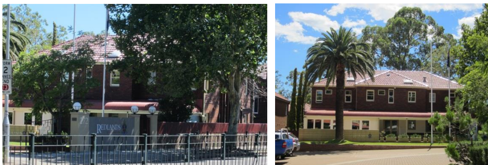
Figure 16 – Located at Military Road, the main entry to Redlands, is the Administrative Office, known as Lone Oak, on the east (left) and the Administrative Office on the west (right) (Source: NBRSPARTNERS, December 2013)
