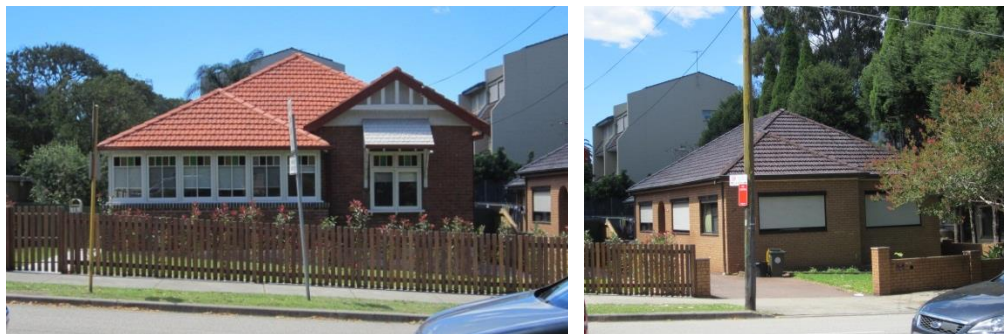
Figure 26 – View to No 15 Gerard Street, residence located at the corner of Winnie and Gerard Streets (left). View east showing Nos 13 and 15 Gerard Street, residential cottages adjoining Redlands (right) (Source: NBRSPARTNERS, December 2013)
