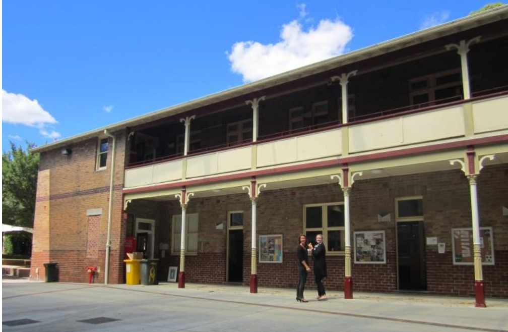
Figure 32 – Liggins Building, two-storey classroom block with verandah located on the eastern side of the building (Source: NBRSPARTNERS, December 2013)
