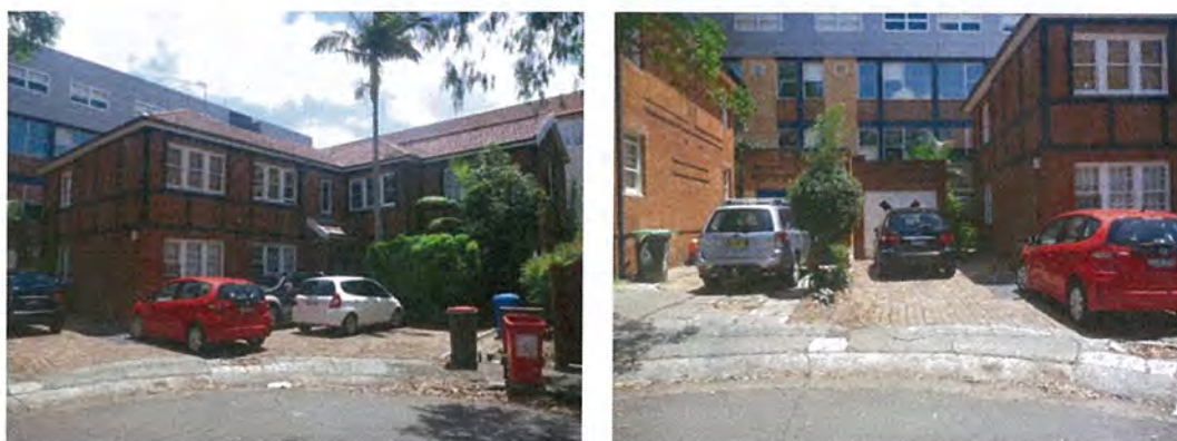
Plate 8.5 View of 7 Monford Place and its associated lock up garage. The building behind the garages is the Roseby Building.
