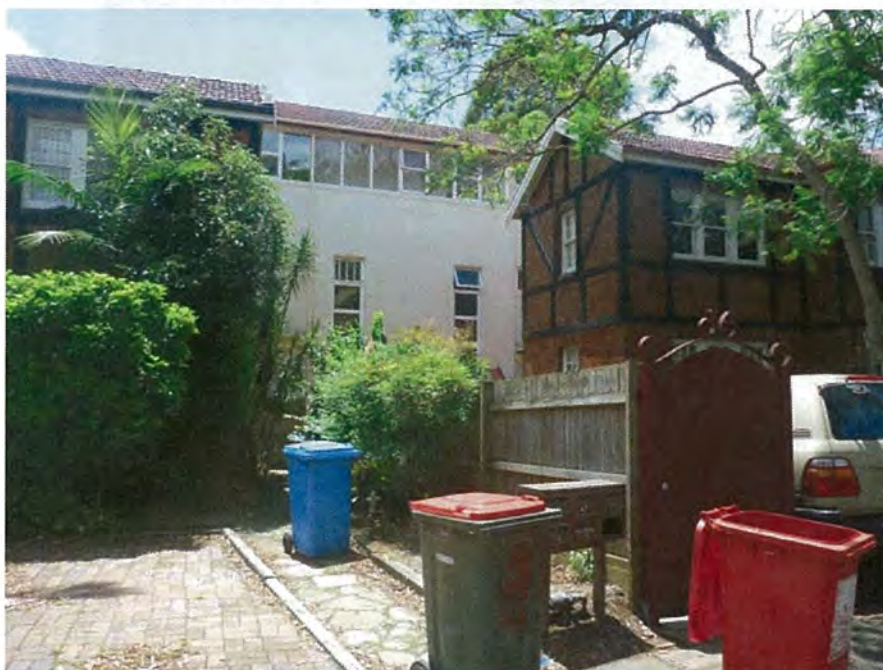
Plate 8.7 View north between 7 and 8 Monford place towards the Mowll Building. A brick-paved, fenced passageway leads between the flats to the Mowll Building; this is shown by the brown fence and maroon gate.
