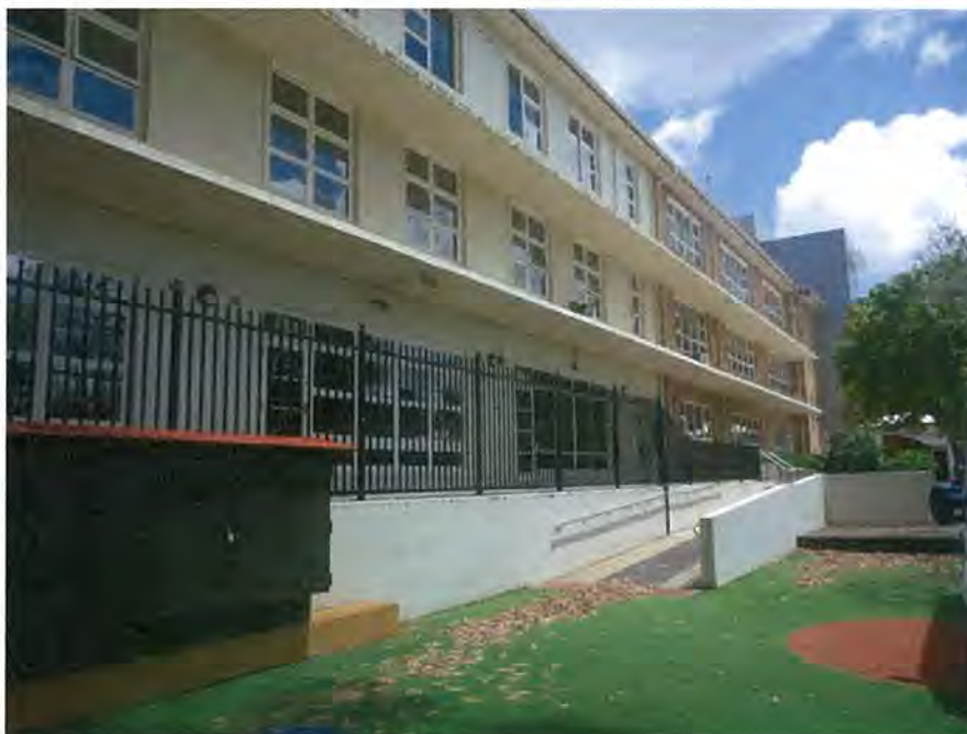
Plate 8.1 South-west facing view of the Mowll Building. The building has undergone multiple phases of additions, with the exposed brick at the far end of the structure representing one such expansion.
