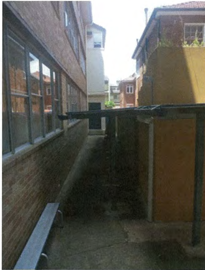
Plate 8.2 View of the walkway at rear (southern face) of the Mowll Building. The brick apartment buildings to the right are 7 and 8 Monford Place. Note the levelled area between structures.
