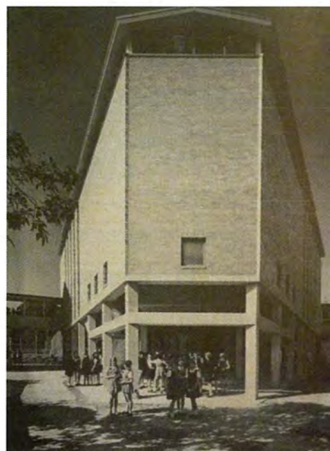
Figure 5.20. The newly completed Assembly Hall c. 1966. (Photograph by Max Dupain in Gillham, Myrtle & Dunlop 1990:222).
