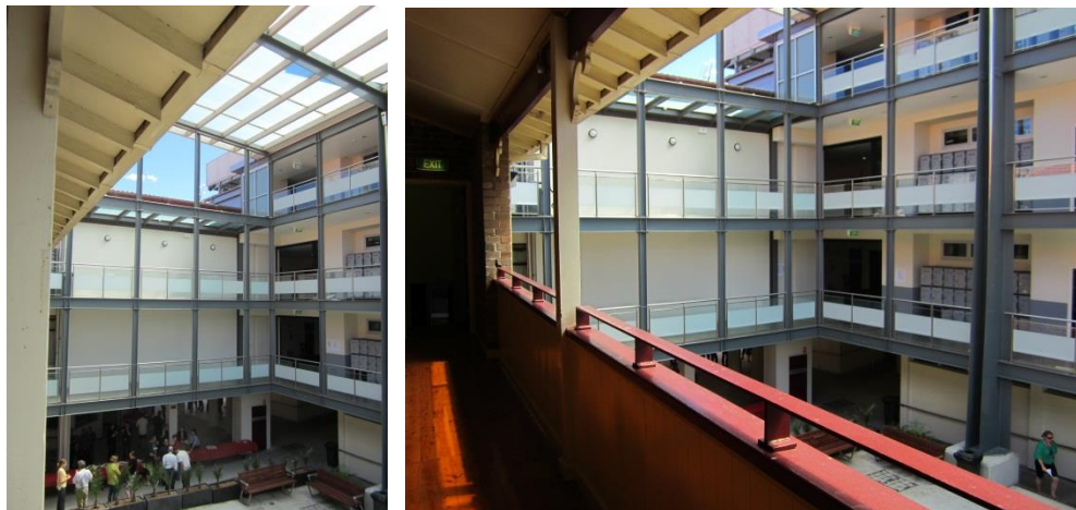
Figure 38 – "Roseby" (formerly Wyndham Building) four-storey classroom block, as viewed from first floor verandah of Liggins Building (Source: NBRSPARTNERS, December 2013)
