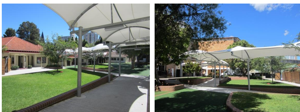
Figure 40 – Courtyard and play areas located north of Mowll Building and south of former Gerard Street cottages with recently constructed shade-cloth (Source: NBRSPARTNERS, December 2013)
