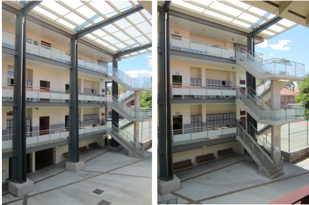
Figure 37 – "Roseby" (formerly Wyndham Building) four-storey classroom block located on the eastern side of Liggins Quad (Source: NBRSPARTNERS, December 2013)
