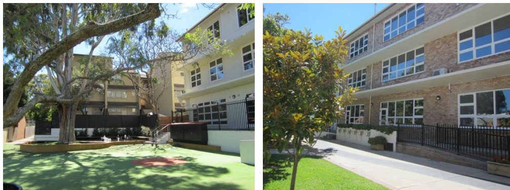
Figure 39 – Mowll Building, North Elevation, three-storey classroom block facing onto courtyard with tree plantings (Source: NBRSPARTNERS, December 2013)
