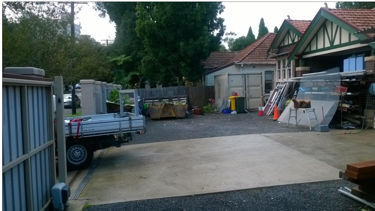
Plate 6: the northern section of the site viewed facing north-east, with Gerard Street to the left.
