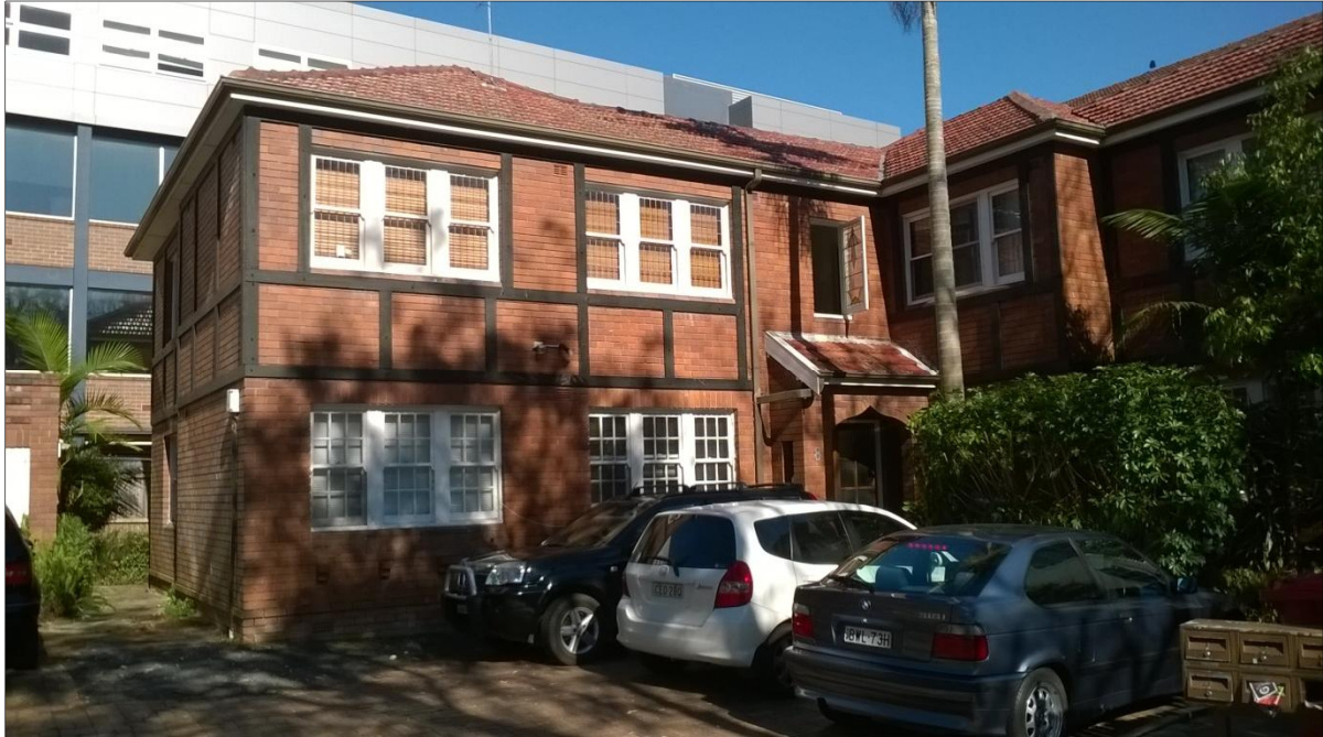
Plate 2: 8 Monford Place in the south-western section of the site.
