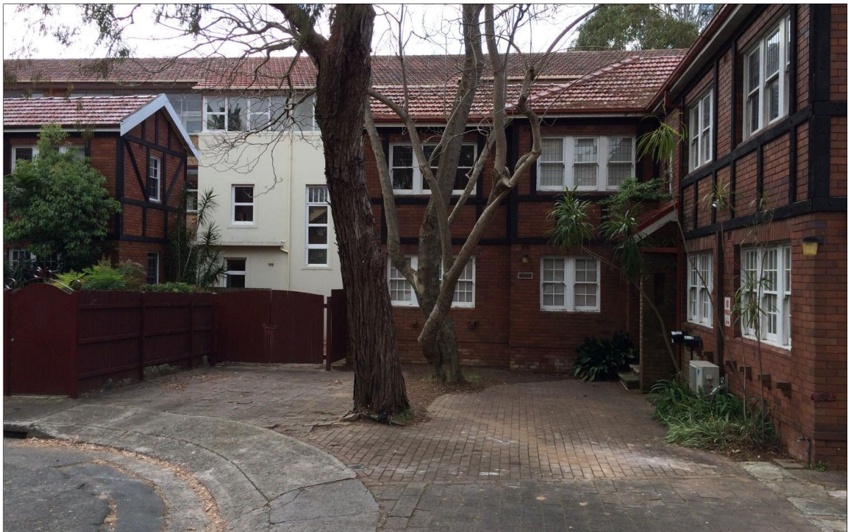
Plate 4: 7 Monford Place in the southern section of the site.
