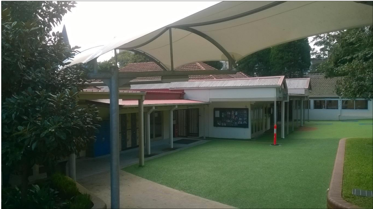
Plate 7: former residential houses now used as school buildings in the northern section of the site.
