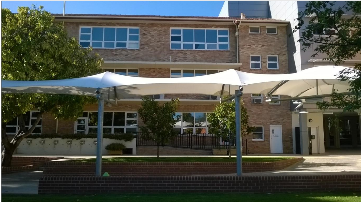
Plate 1: The Mowll Building in the centre of the site.
