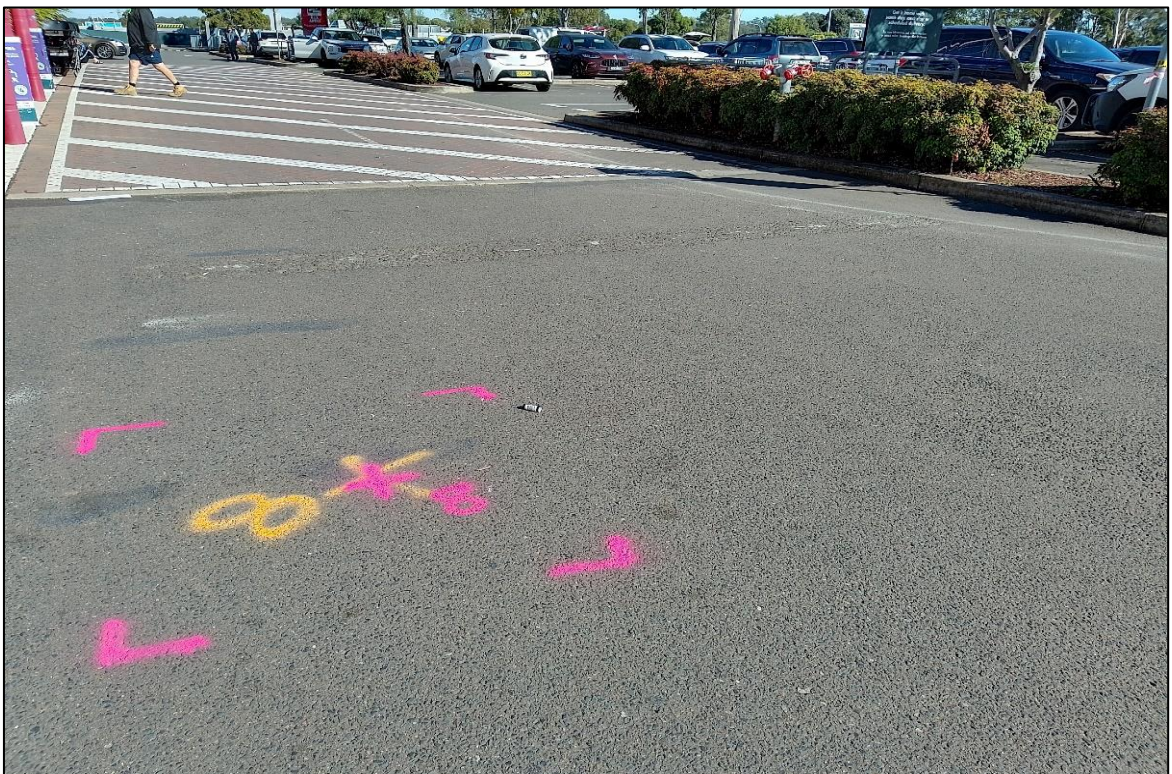
Photograph 22 - General vicinity of BH8.
