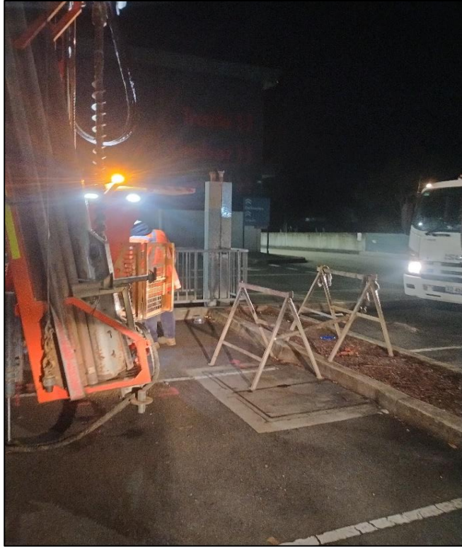
Photograph 25 - General vicinity of BH10.
