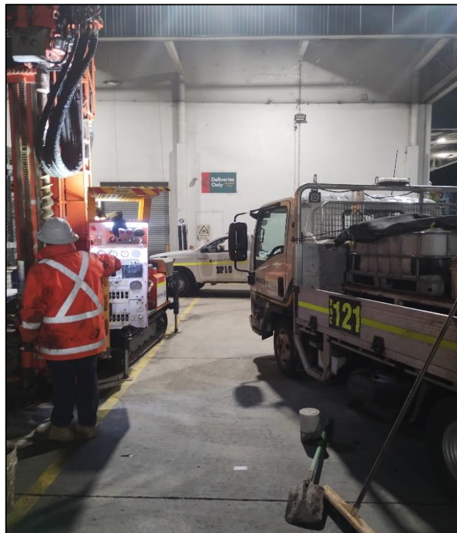
Photograph 14 - General vicinity of BH2A.
