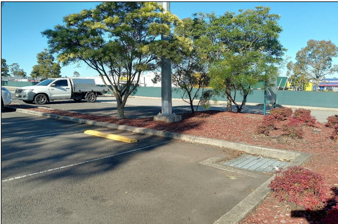
Photograph 4 - Garden beds in carpark area in north western portions of the site.
