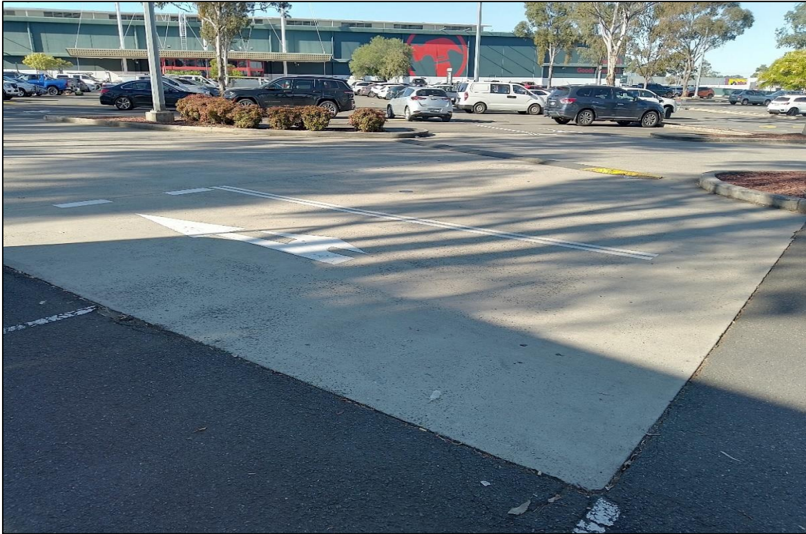
Photograph 3 - Sealed concrete within north western portion of the site.
