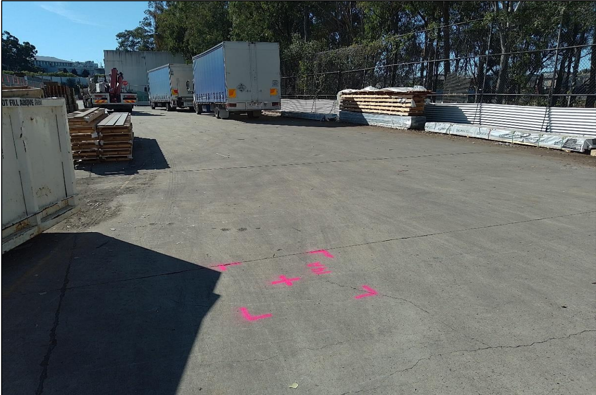
Photograph 31 - General vicinity of BH14A.
