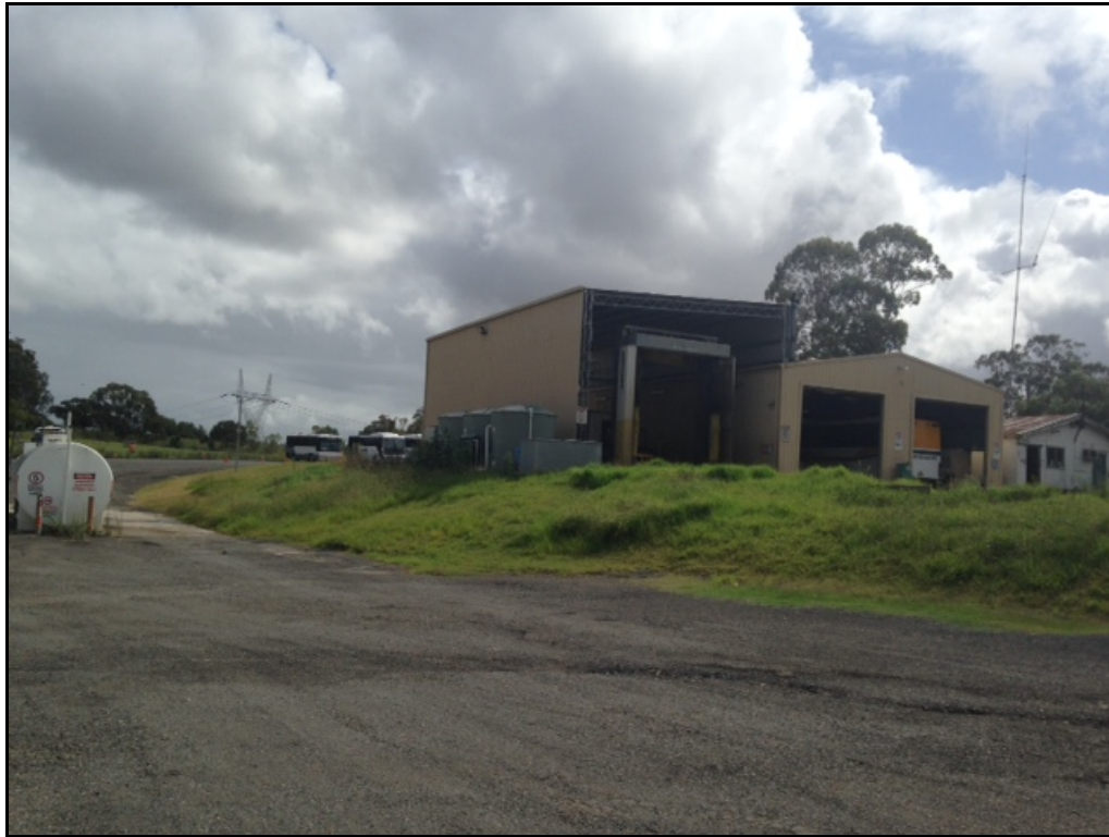
Plate 7: The bus depot and associated infrastructure. Photograph taken looking north-east.
