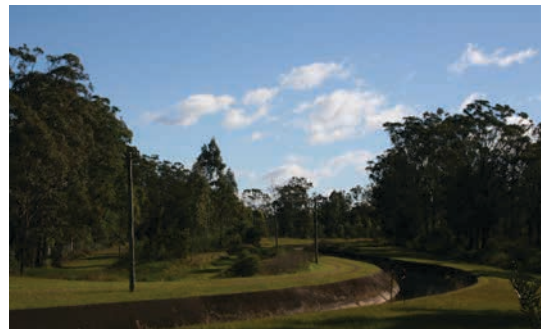
4. Upper Canal System to the west of the site
