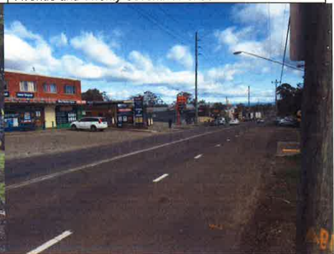
Figure 6 – Existing centre at Fifteenth Avenue
