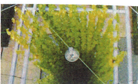
2. Tensioned wires with climber
