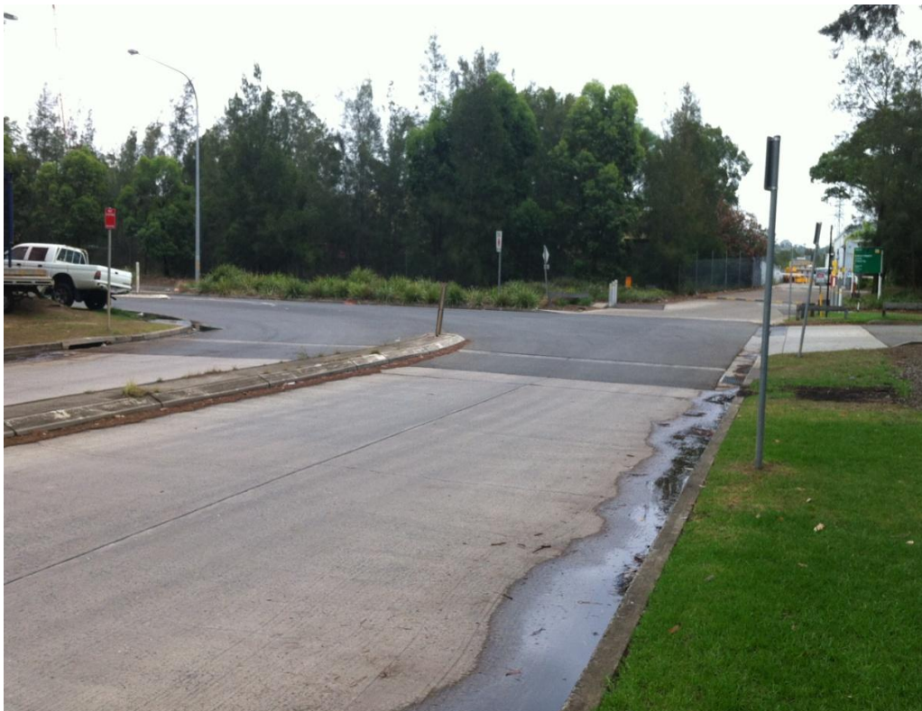
Figure 7: Existing intersection of Burroway Road and Hill Road, looking west
