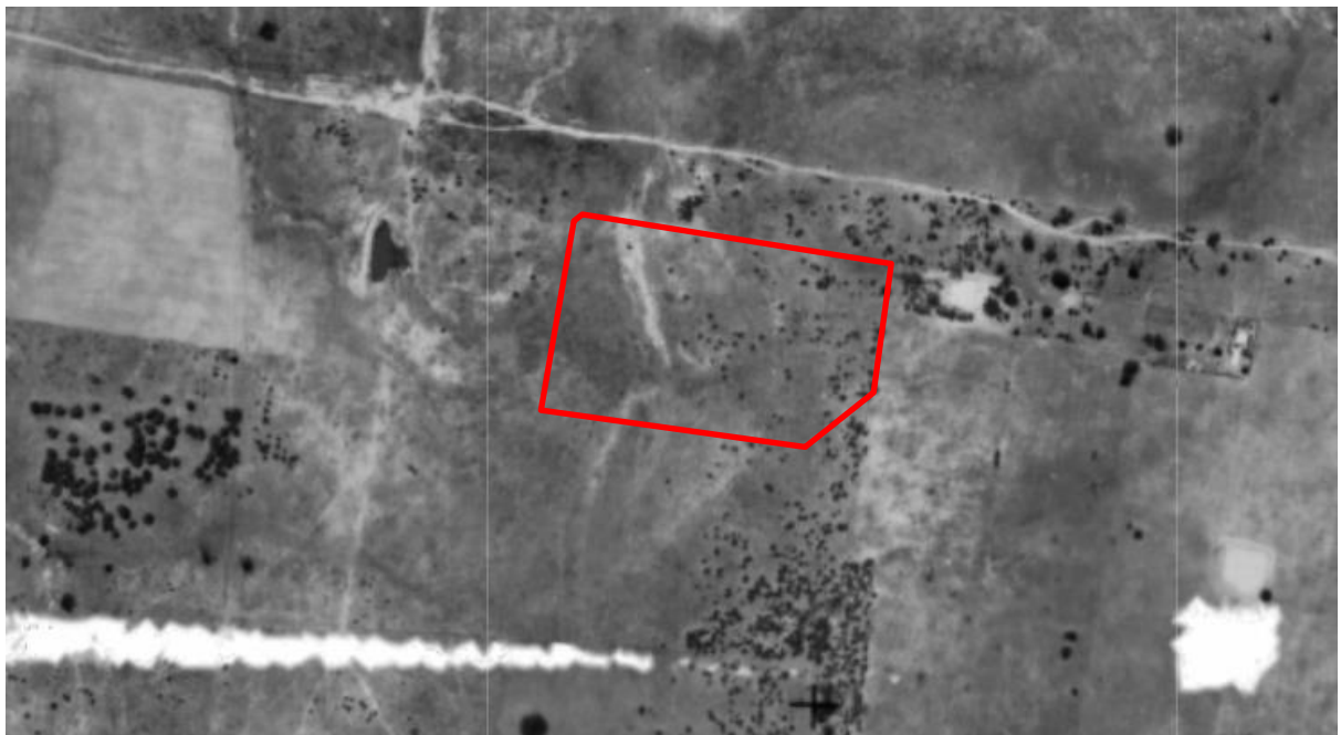
Figure 10 – c.1947 aerial image of the subject site within the context of its immediate locality.
