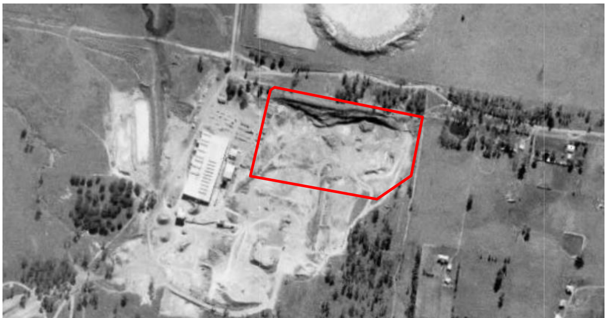
Figure 12 – c.1975 aerial image of the subject site within the context of its immediate locality.
