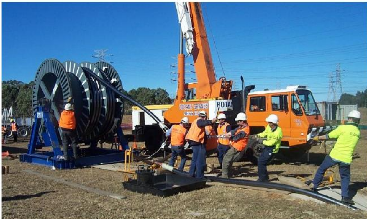
Figure 4-26 Cable pulling
