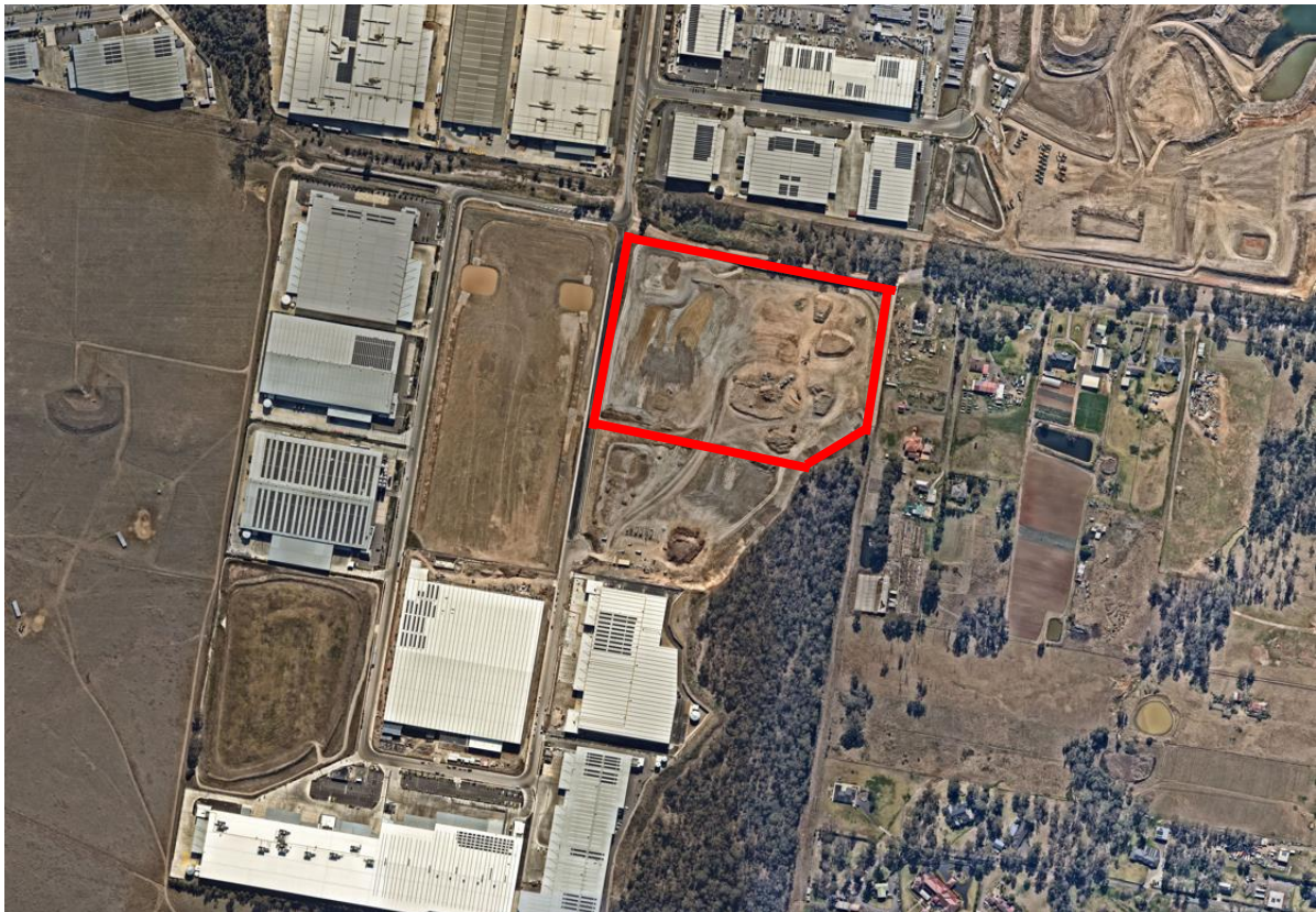
Figure 1: Site Aerial Photograph (Proposed Lot 305 - Development Site). Source: Nearmap (2023)
