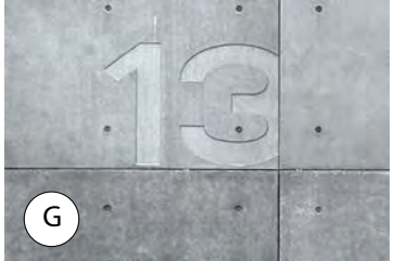
POLISHED CONCRETE PANELS CAST ON SITE TFD
