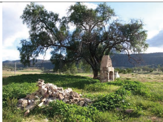
Plate 28 Cottage Chimney Remains and piled sandstone (c.1930)
