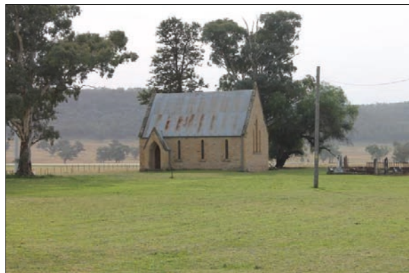
Plate 4 Bylong St Stephen's Anglican Church (c. 1876)
