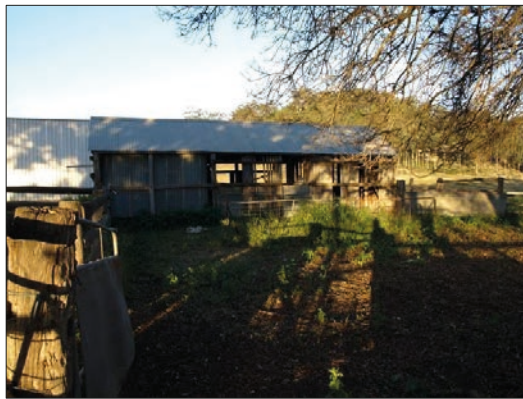
Plate 15 Bridgelo Provisional School (c. 1915)
