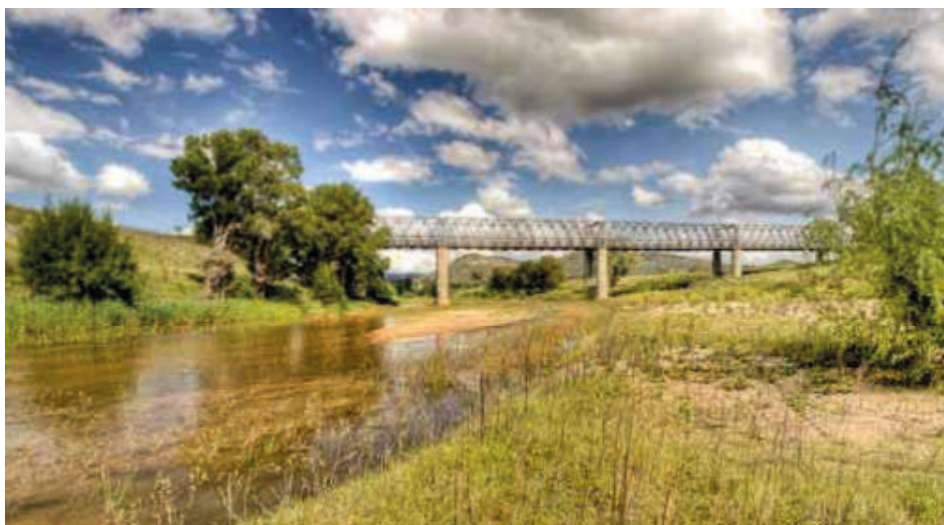
Bylong Valley – Bridge over the Goulburn River
