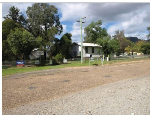
Plate 12 Bylong Upper Public School: building 2 (c. 1975)
