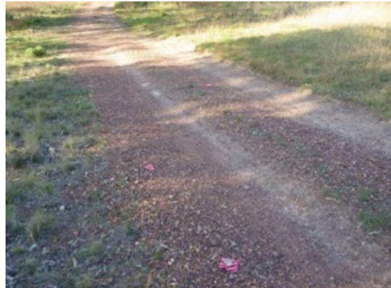
Plate 4 Example of ground surface and track at RPS 027
