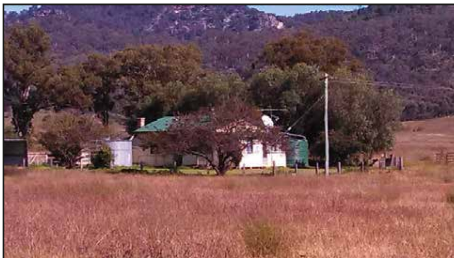
Print 1 Valley View– external walls are ACM.
