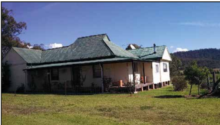
Print 22 Dwelling opposite the school within the Eastern Open Cut Mining Area. Likely to contain asbestos within the wet areas of the dwelling.
