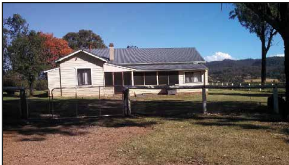
Print 15 Part of the accommodation area.
