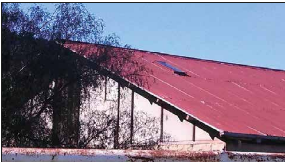
Print 18 One of the Tarwyn Park Sheds with ACM.
