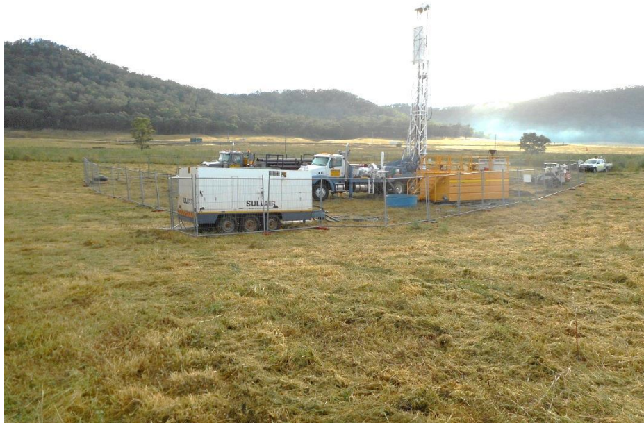
Figure 4-6 Drilling at Test Site 1
