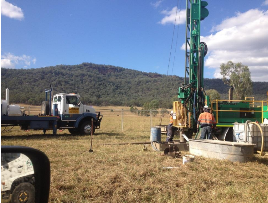
Figure 4-7 Drilling Test Site 2 east of Bylong River
