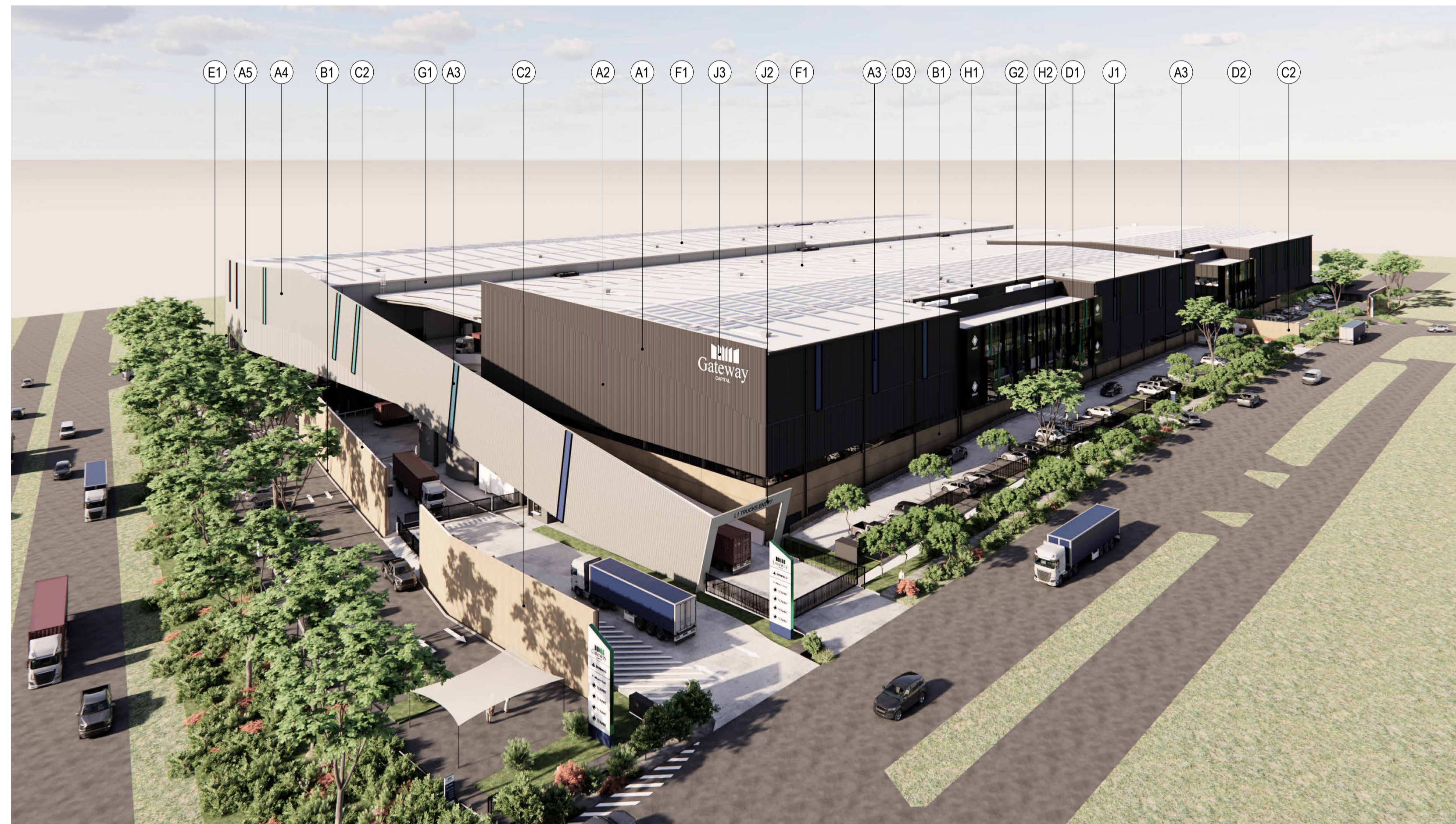
H1 ALUMINIUM WINDOW SHROUD TO WAREHOUSE EXTERNAL WALL (APPROX 6-10mm THICK x 300-400mm DEEP) BLACK
