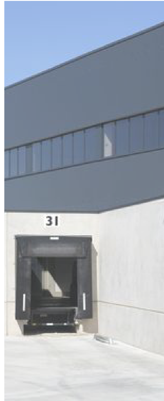
Horizontal clear glazing to warehouse facade
