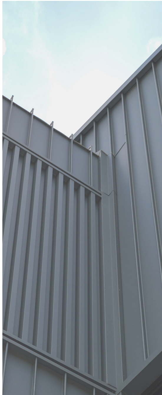
Standing seam cladding - warehouse facade
