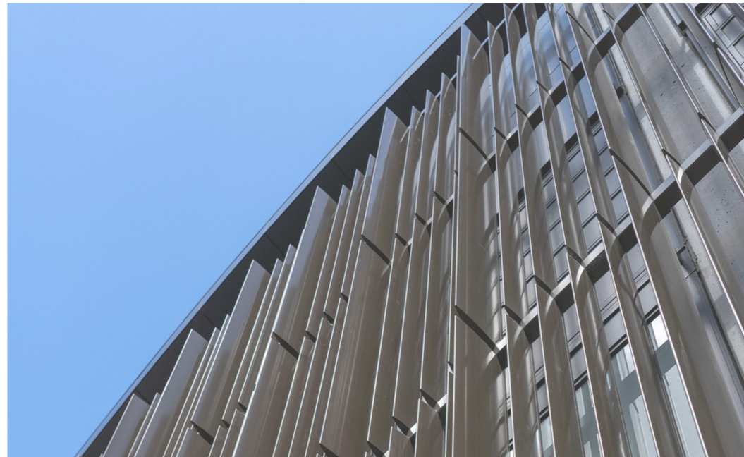
Glazed office facade with vertical battens
