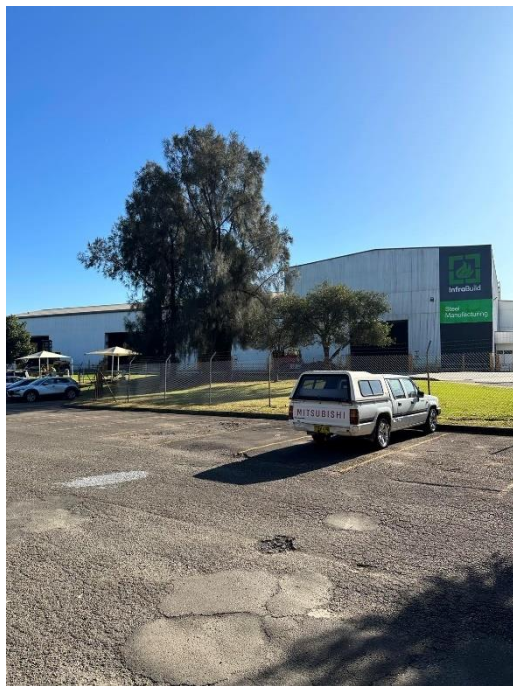
Picture 4 View of existing industrial building
