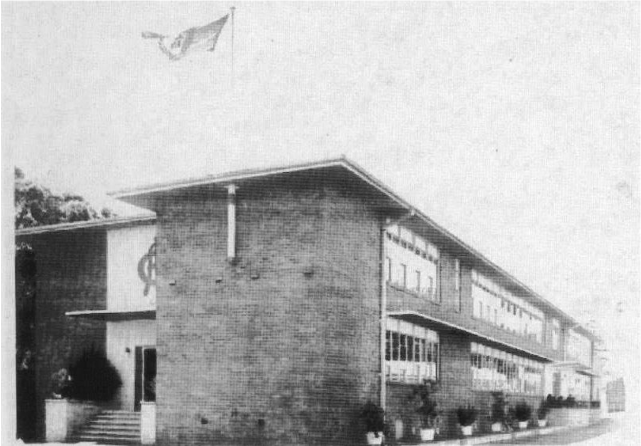
Figure 21 - New Robertson & Marks-designed Administration building, 1962.
