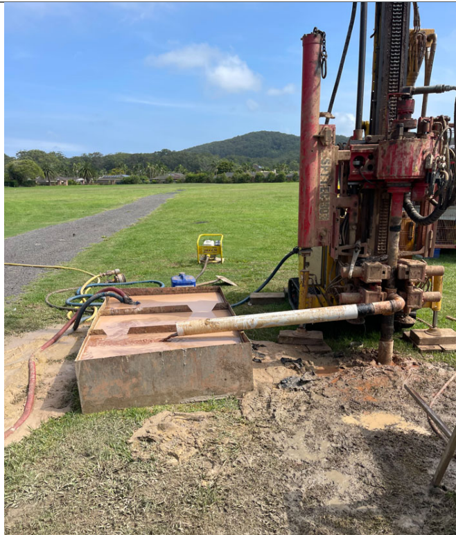
IMAGE 6 – Ongoing drilling at BH10.
