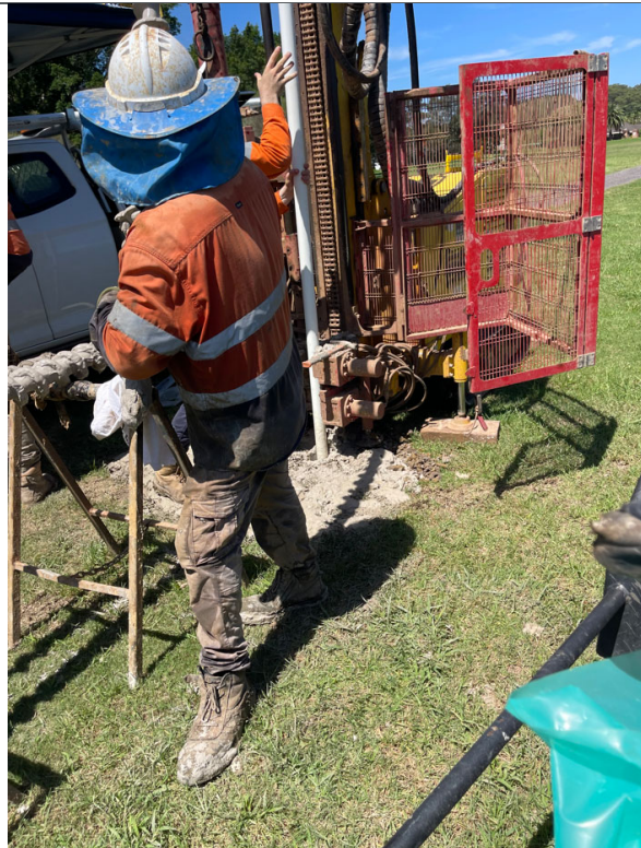
IMAGE 7 – Installation of PVC pipe in one of the groundwater monitoring bores.
