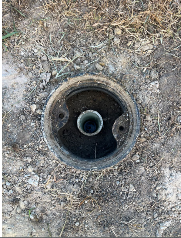
IMAGE 9 – Installed piezometer during groundwater testing and sampling.
